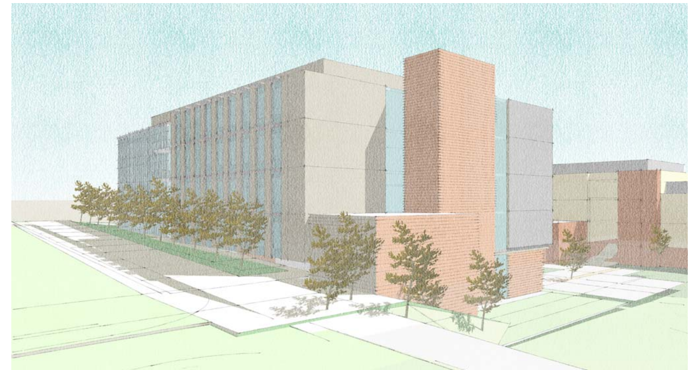
Looking Southeast from the Pedestrian Walkway
