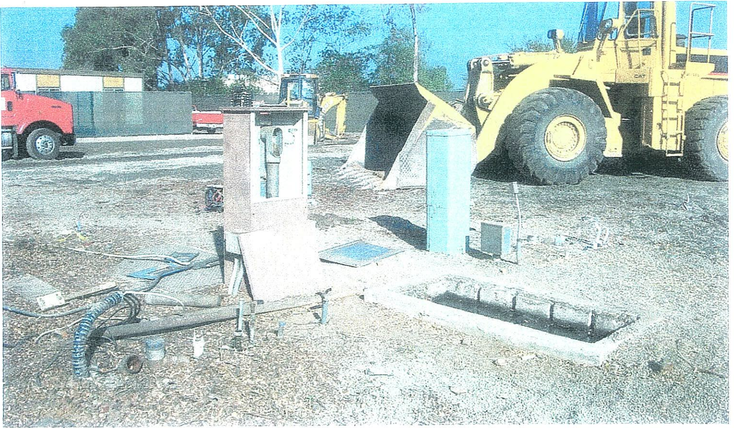
Photograph 5. Utilities at Project Site.
