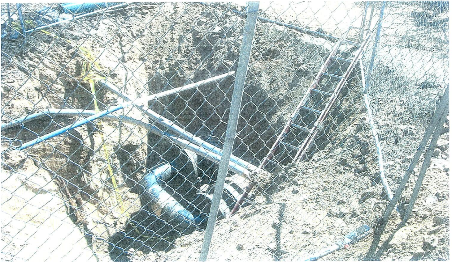
Photograph 6. Water Connection at Project Site.
