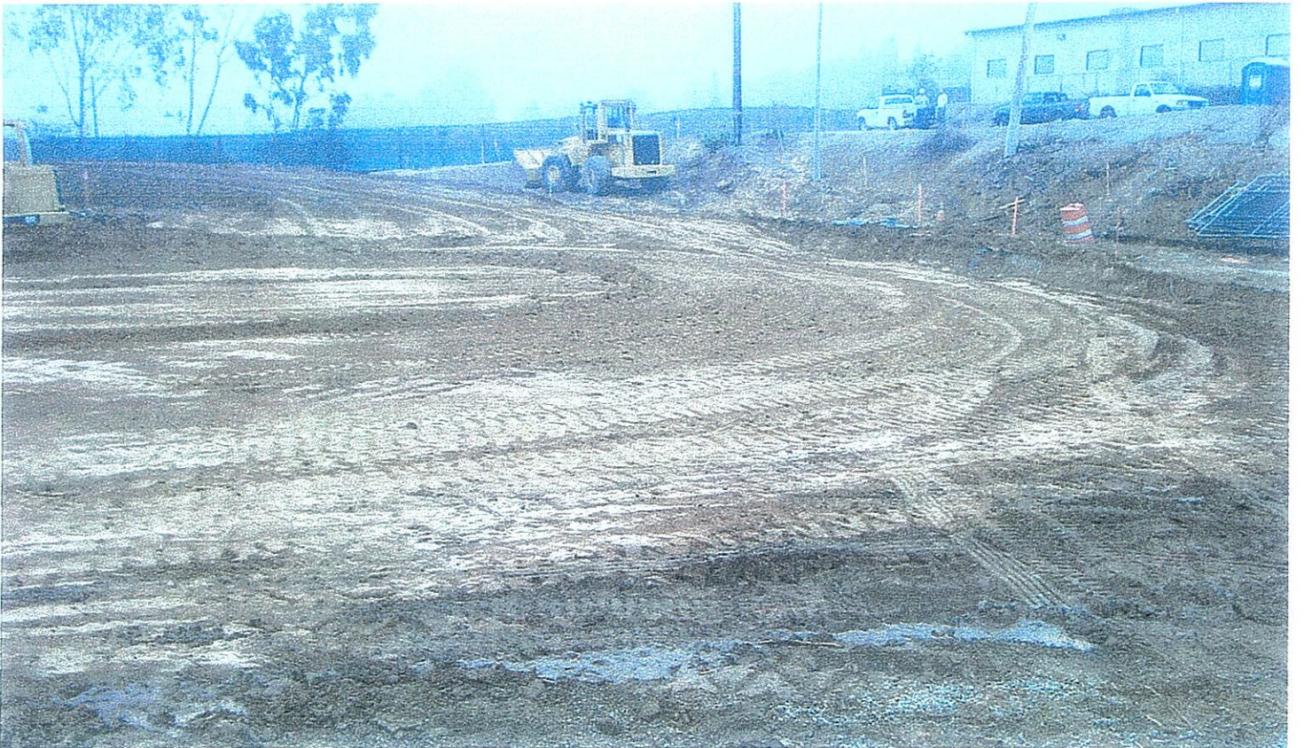
Photograph 12. Grading in Area of Chiller Plant (SE).
