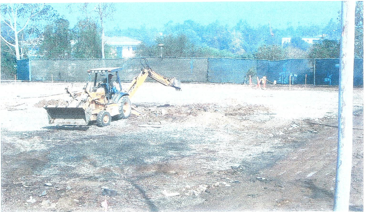
Photograph 9. Breaking Up Apshalt.
