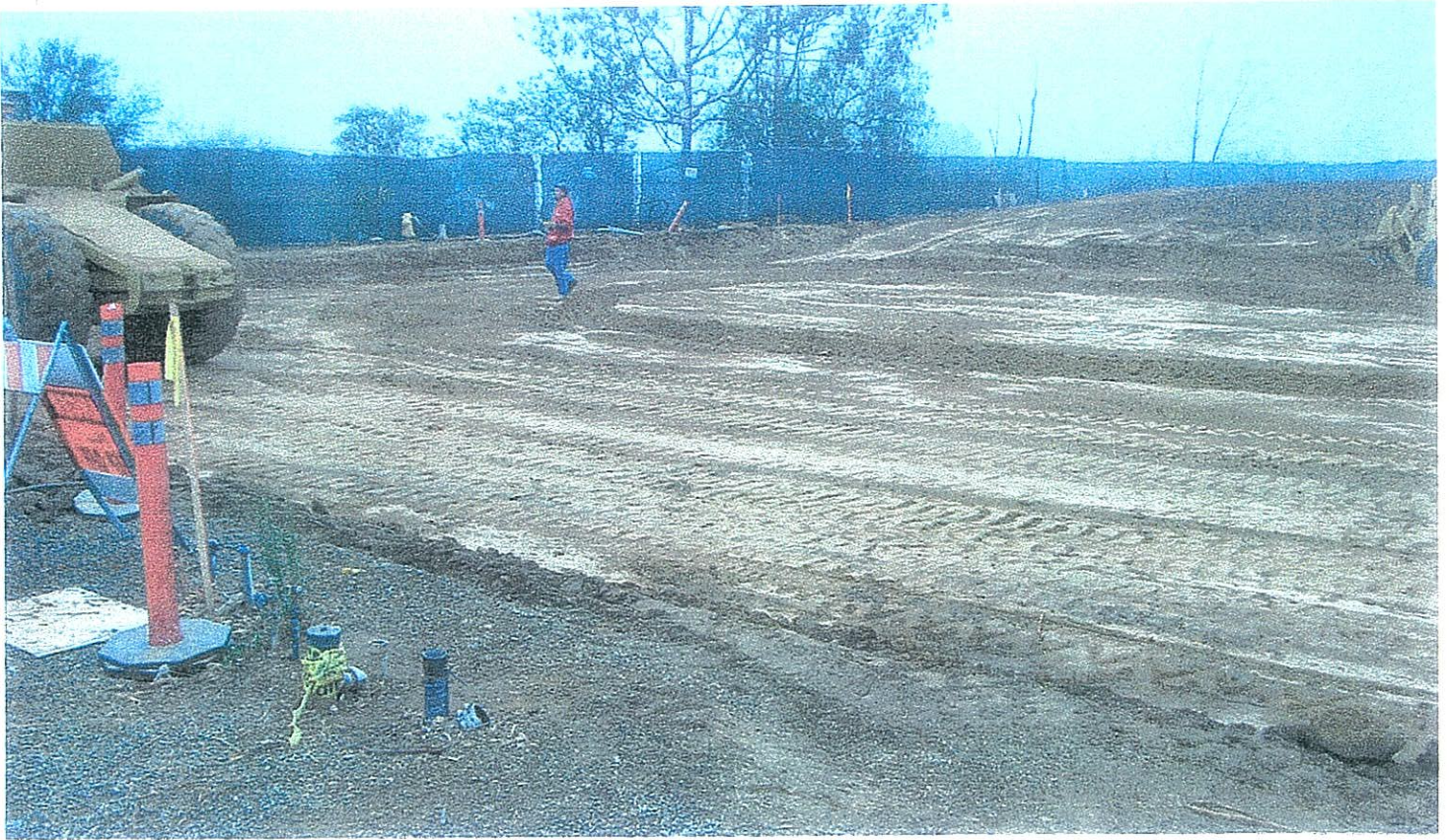
Photograph 15. Overview to SE.
