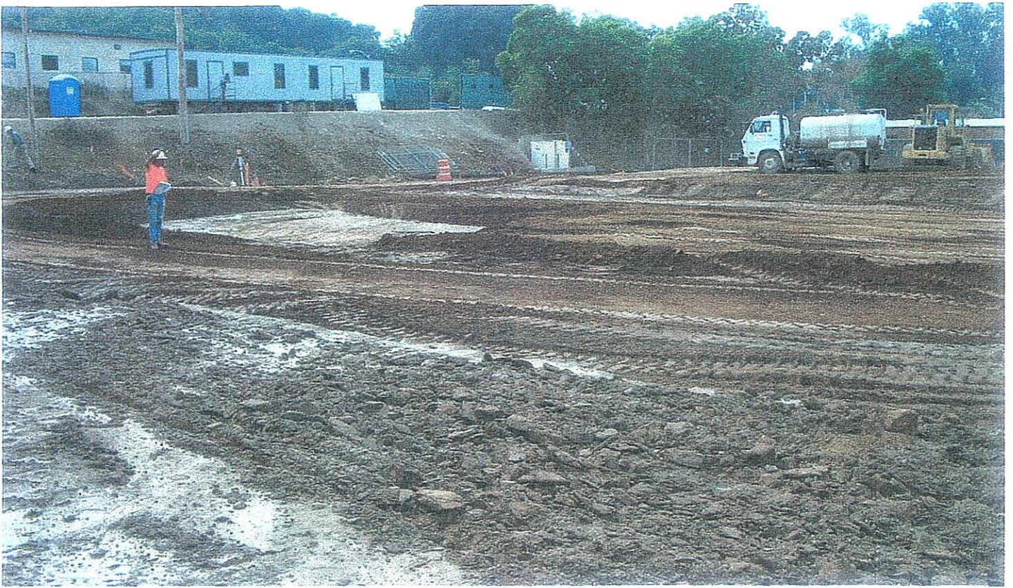
Photograph 21. Overview to Southwest.
