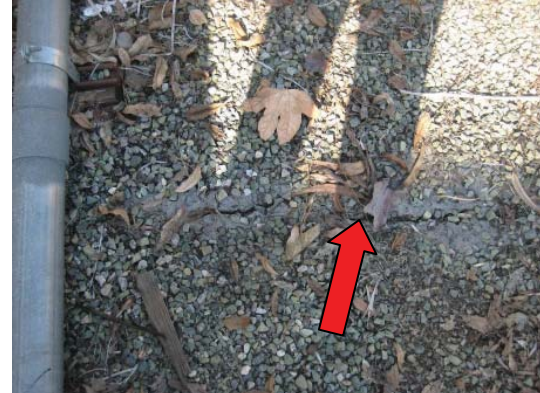
Photo 17 Crack (arrow) in the roofing membrane over the expansion joint in the corridor between Building B and Building C
