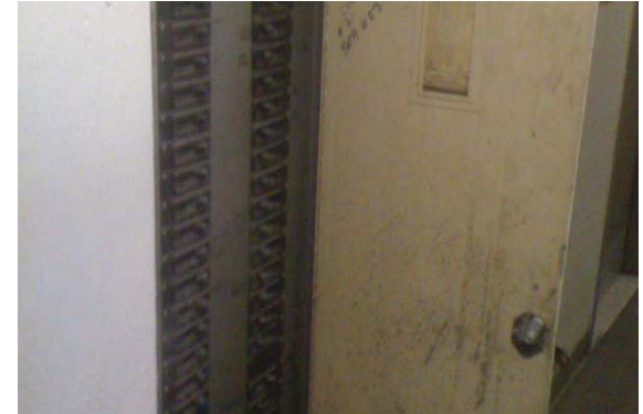
Figure 21 - Typical Building Panel board
