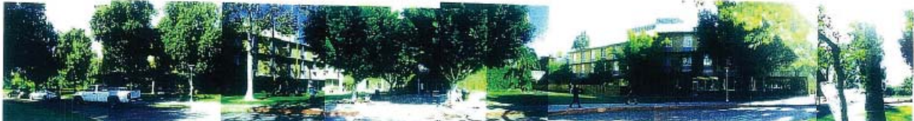
A - I Entry Looking East
