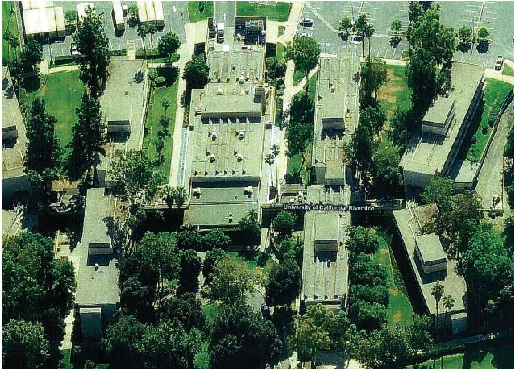
A - I Aerial From the West
