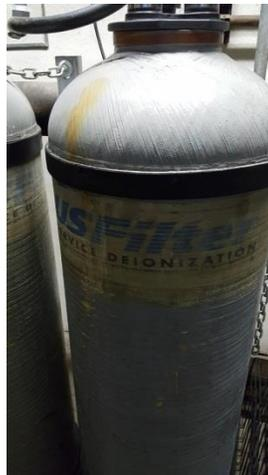
Typical Deionizer system for bank of laboratories
