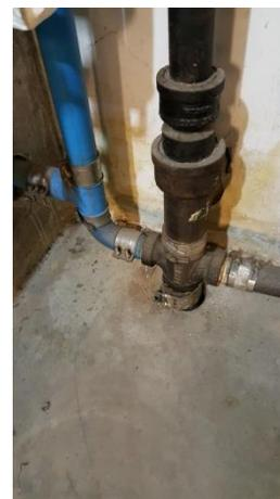
Laboratory waste piped to sanitary waste and vent system using acid waste piping
