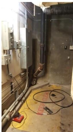
4" and 2" waste and vent stacks at each end of mechanical shaft
