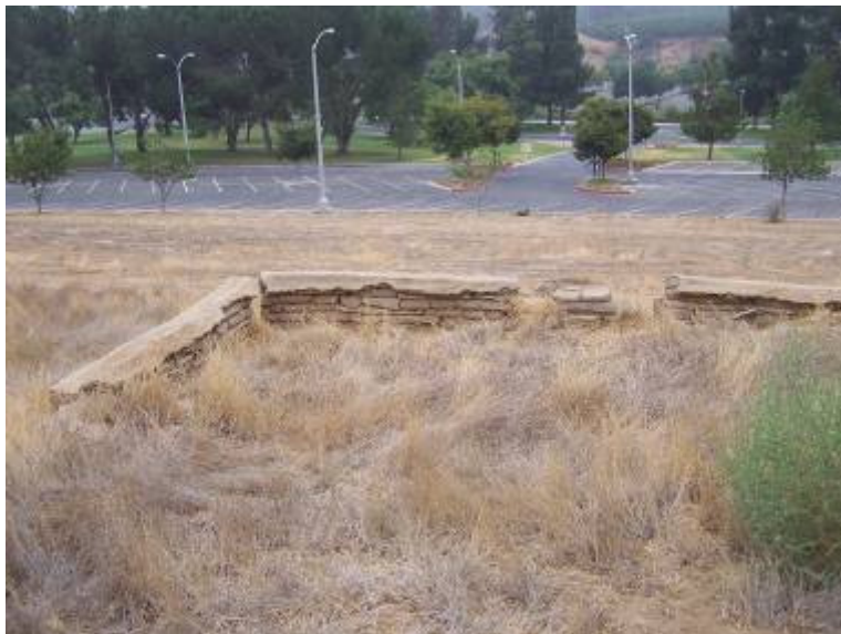
View to south at cesspool structure
