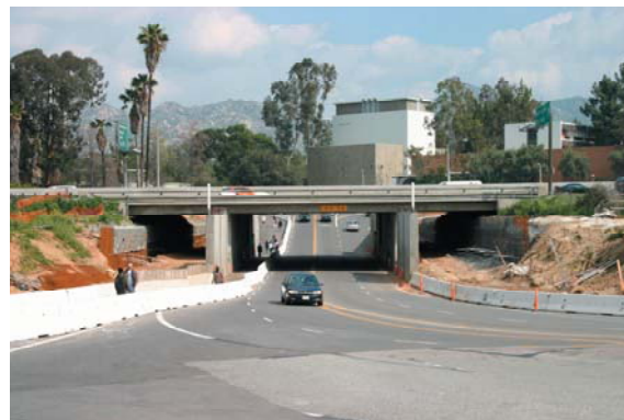
1. Approaching the underpass from West Campus
