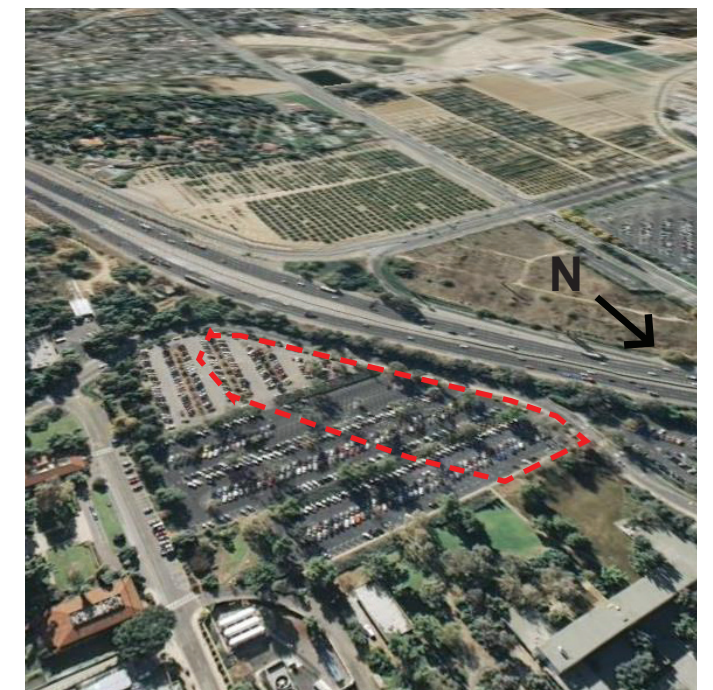
Aerial View From NE
