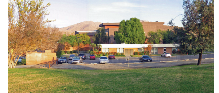
View from Reservoir
