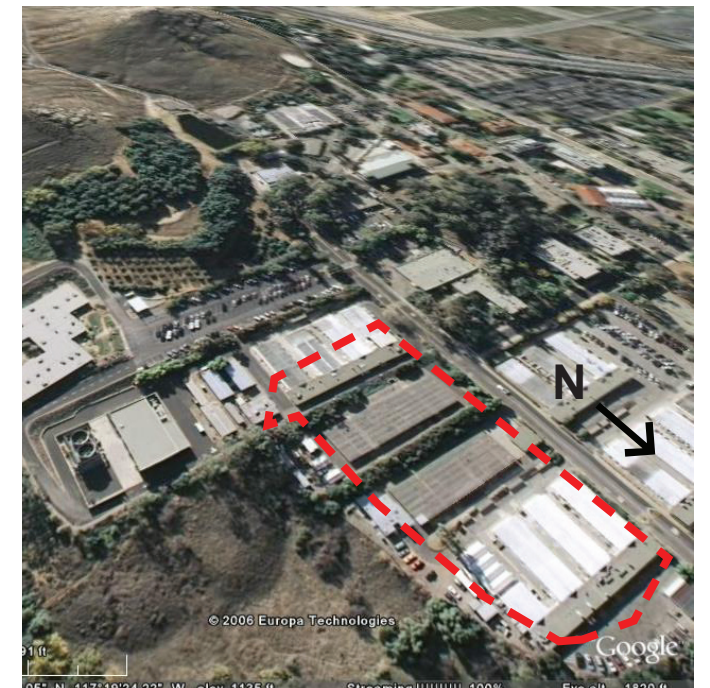
Aerial View From NE
