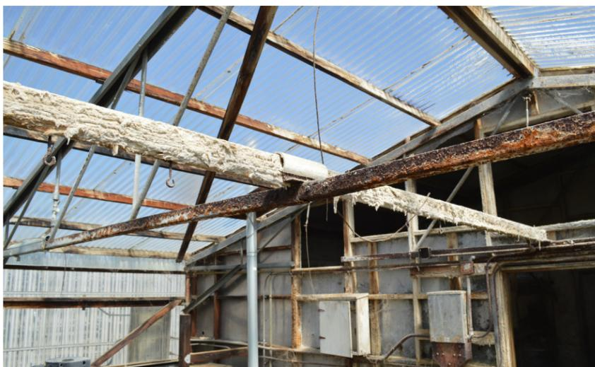
Figure A.4 West Campus. Degrading structure in GH 16-22
