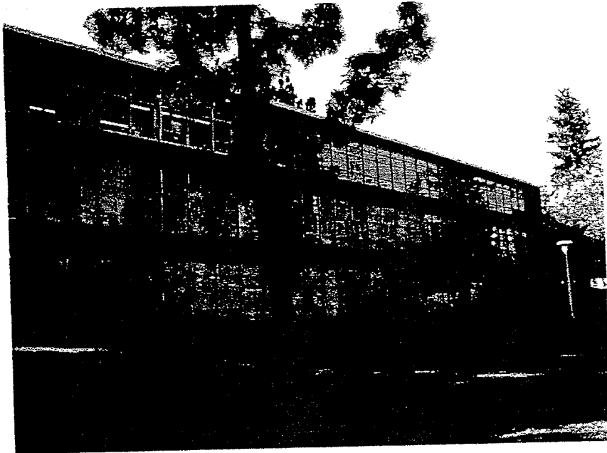
Figure 12: Open North Face of North Building
