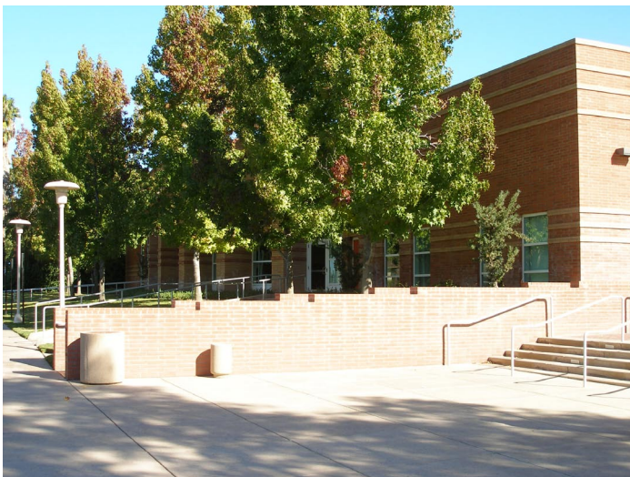
View North Towards Existing Ramp Entrance
