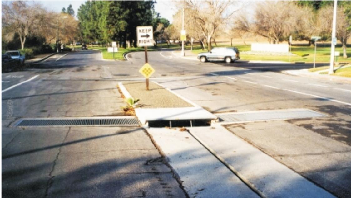
**(4a)** Intake road grates where surface flow conveyed along Big Springs Road enters main 72" campus pipe, view is looking west on Big Springs Road into campus entrance.
