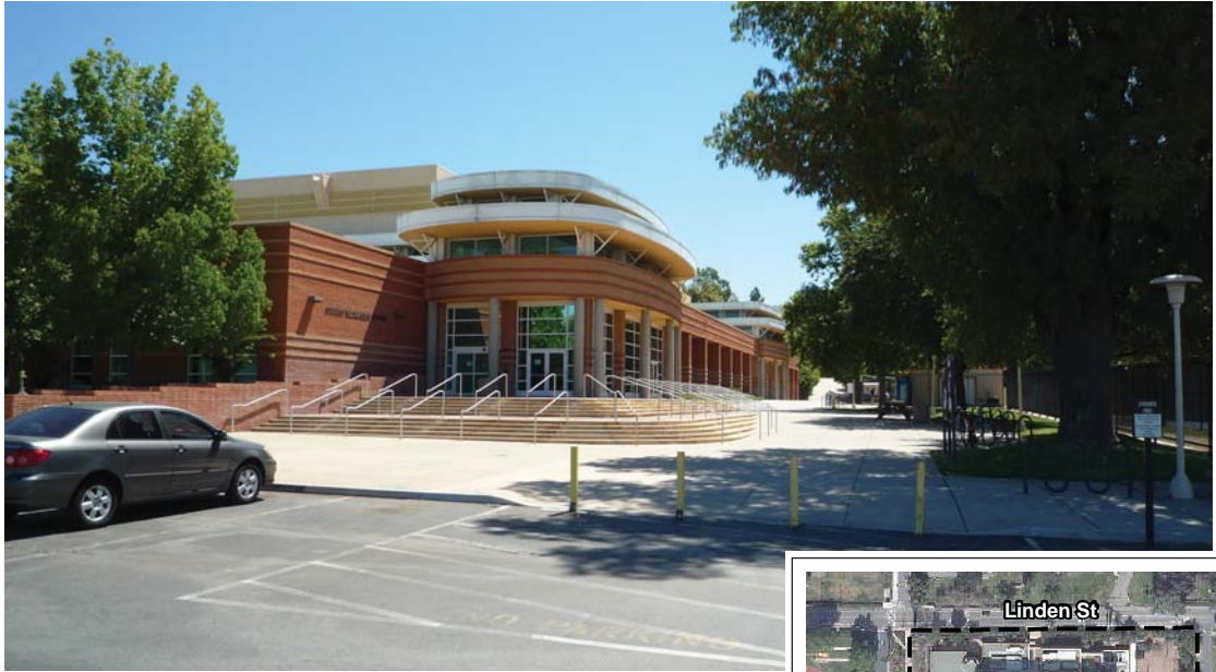
View 1 – View to the east of the existing SRC building.
