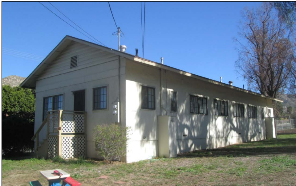
Two-bedroom duplex unit on Blaine Alley.
