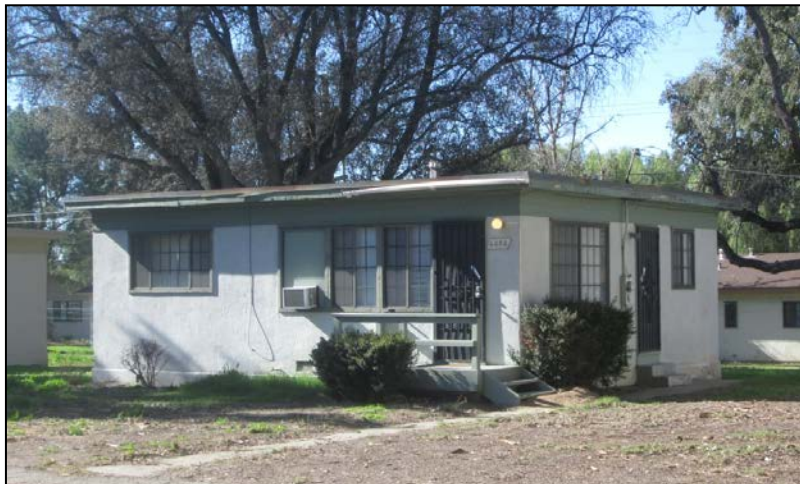
Single unit with original flat roof system on Utah Street.
