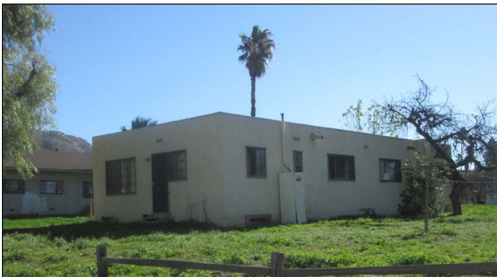
Figure 11: The last remaining duplex unit with pediment walls on Avocado Street.
