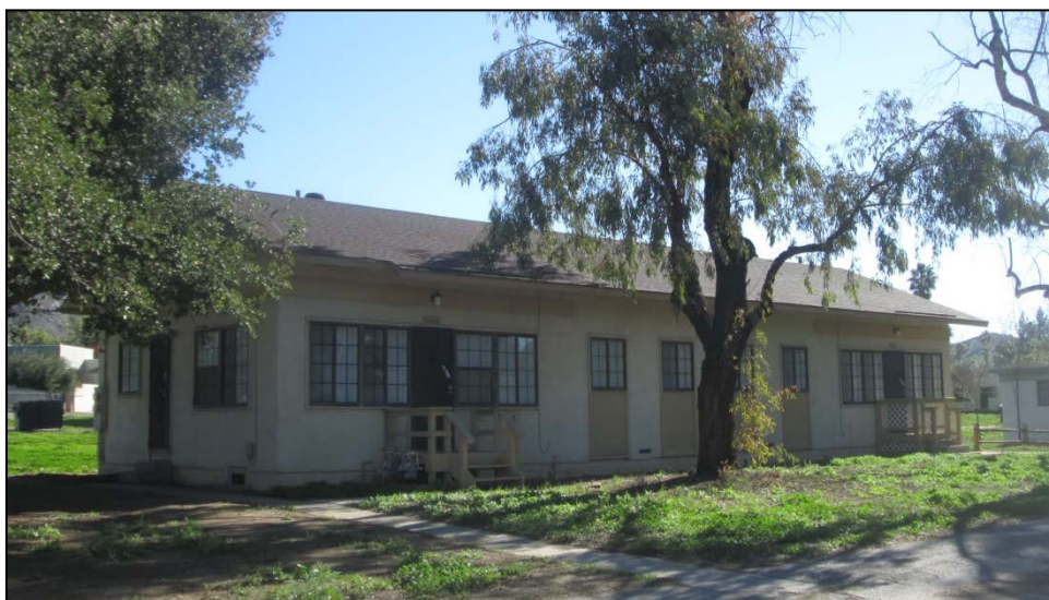
Two-bedroom duplex unit on Utah Street.
