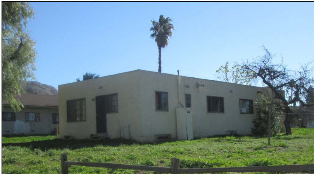
The last remaining duplex unit with pediment walls on Avocado Street.
