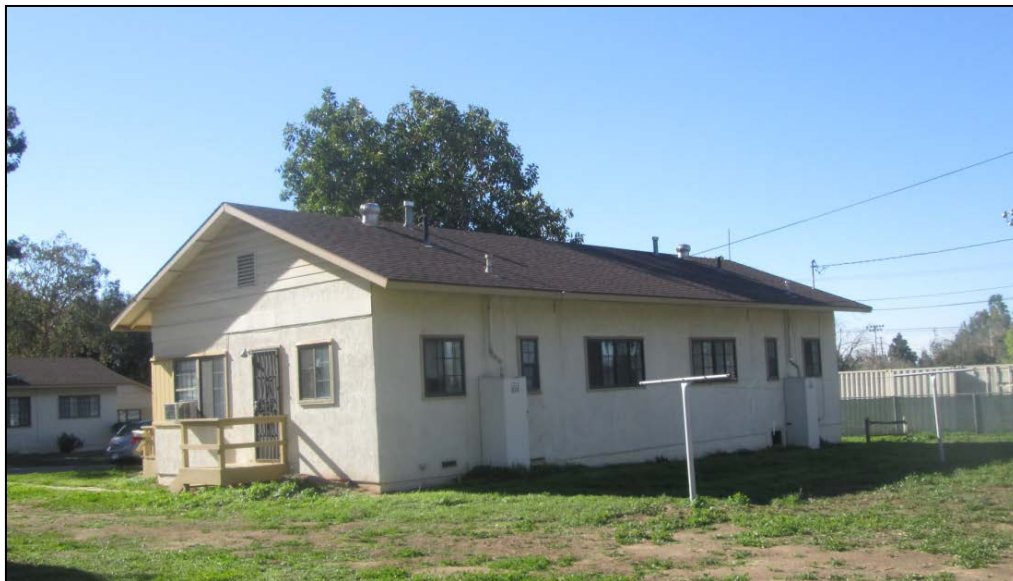
Duplex with replacement gable roof system on Grape Street.
