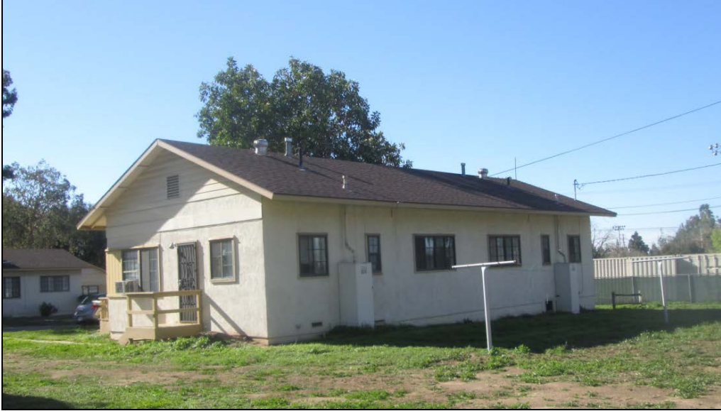
Figure 12: Duplex with replacement gable roof system on Grape Street.
