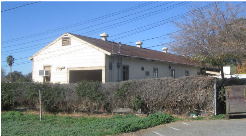
Maintenance yard building (constructed circa 1965) - west of Avocado Street
