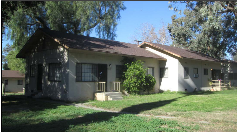
Offset duplex unit on Utah Street.
