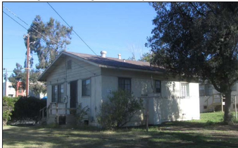
Single unit with replacement roof system on Blaine Alley.
