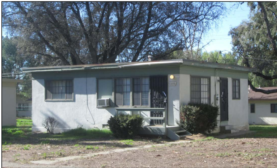
Figure 9: Single unit with original flat roof system on Utah Street.
