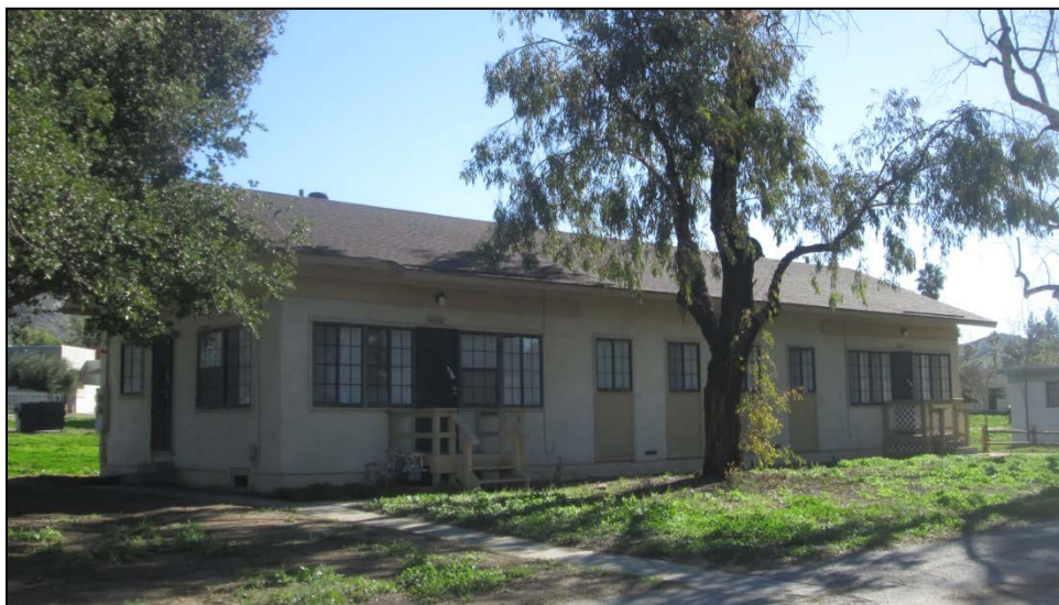
Figure 15: Two-bedroom duplex unit on Utah Street.
