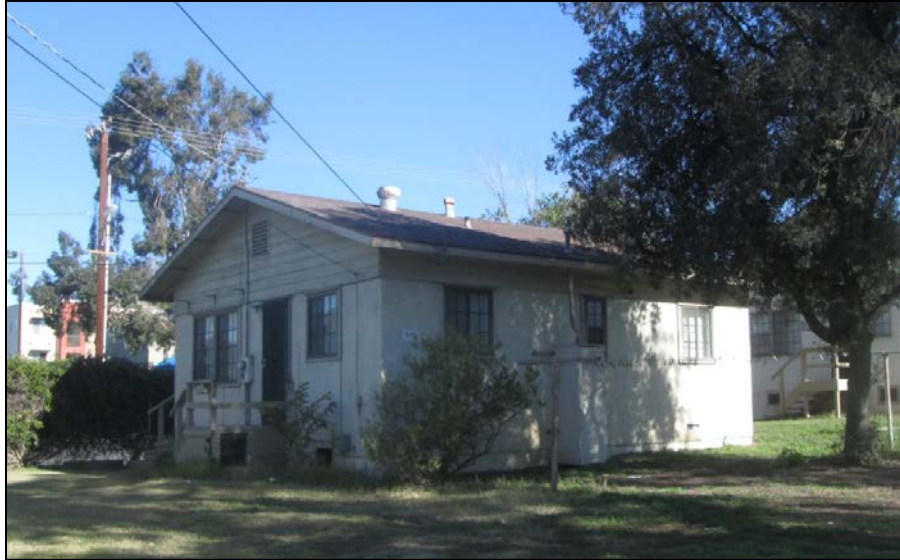
Figure 10: Single unit with replacement gable roof system on Blaine Alley.
