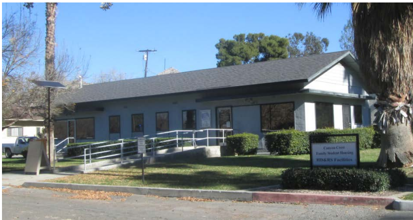
Building that houses Resident Services (constructed circa 1978) - Avocado Street
