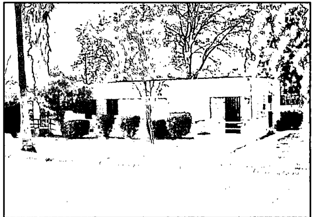
One of the few relatively unaltered buildings in the compound
