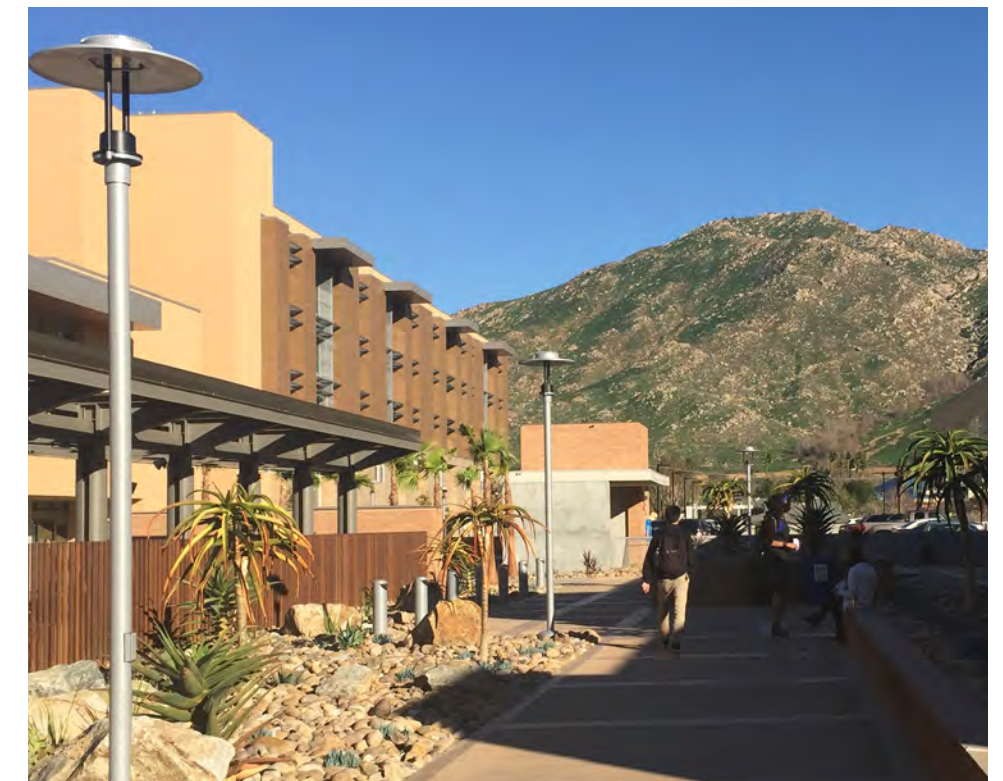
Student residential apartments at Glen Mor
