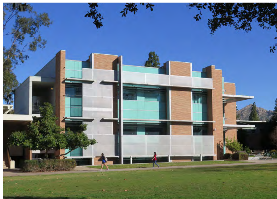
Existing buildings do not present a positive edge to the Carillon Mall
