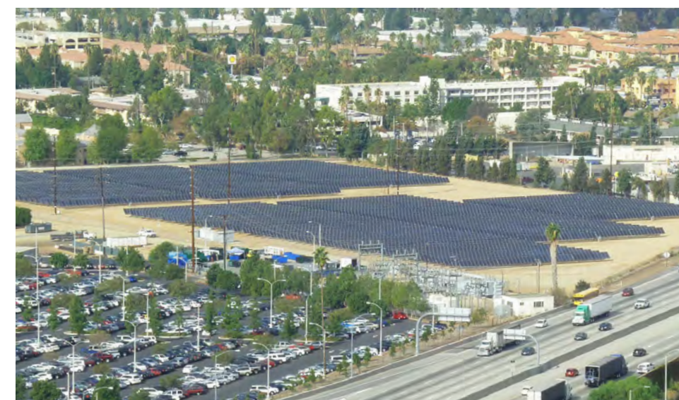
Solar array on West Campus
