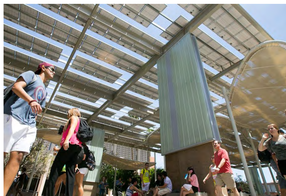
Solar panels create a canopy over public space outside Arizona State University's Memorial Union
