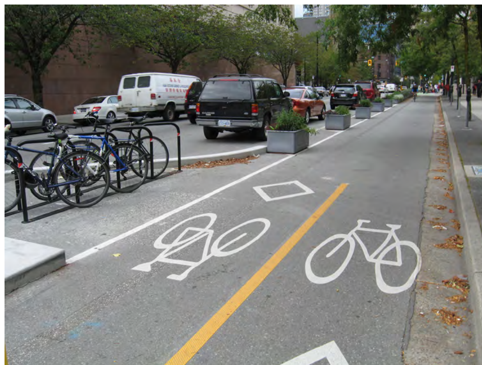
On-street parking, bike corrals, and planter boxes create a protected two-way cycle track, Vancouver B.C.
