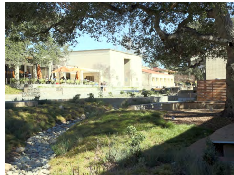
Stormwater swale adjacent to campus building, Claremont McKenna College
