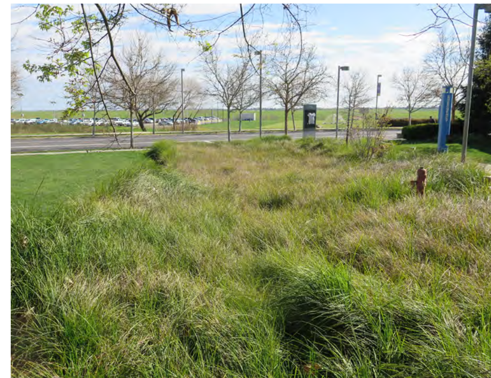
Stormwater swale, UC Merced
