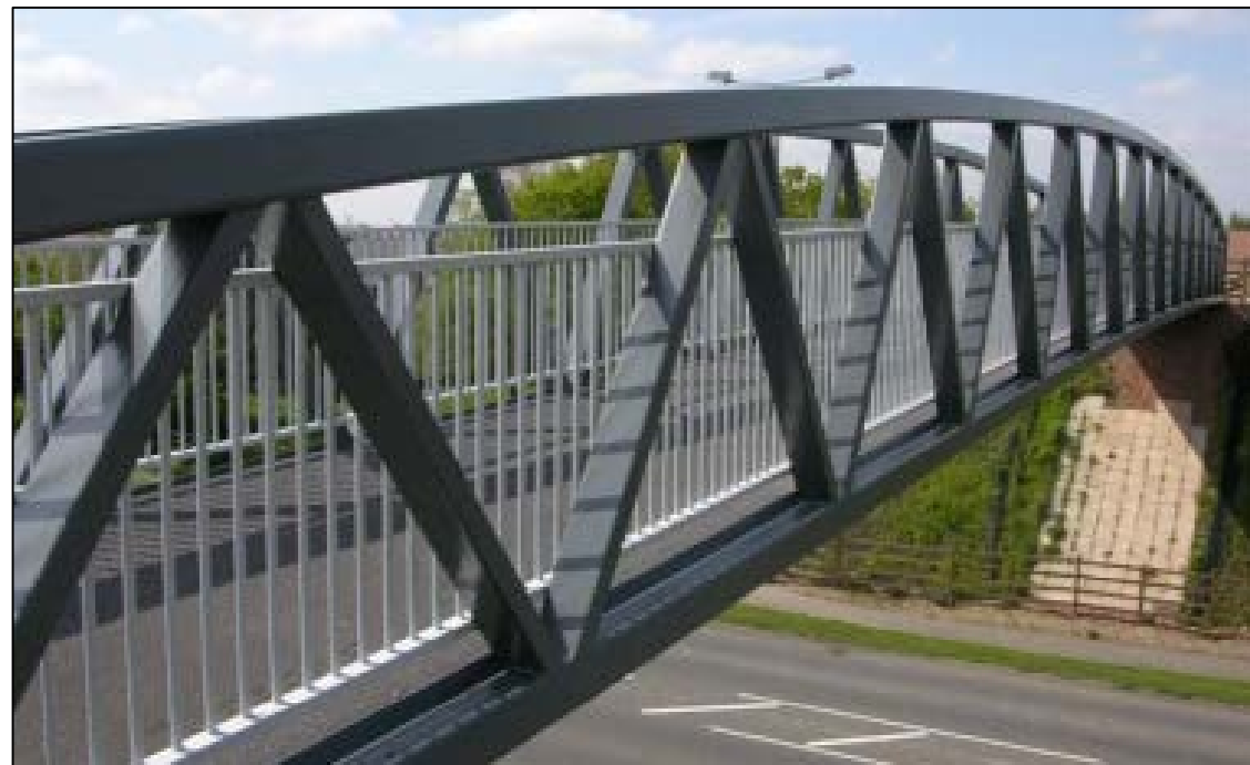
Figure 2.26 – An example of a prefabricated pedestrian bridge at Jades Crossing (Courtesy of NuSteel Structures)
