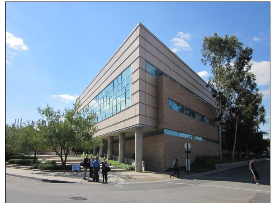
Issue: Disconnected pedestrian path
