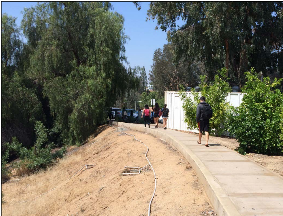
Issue: Unsafe pedestrian path along arroyo
