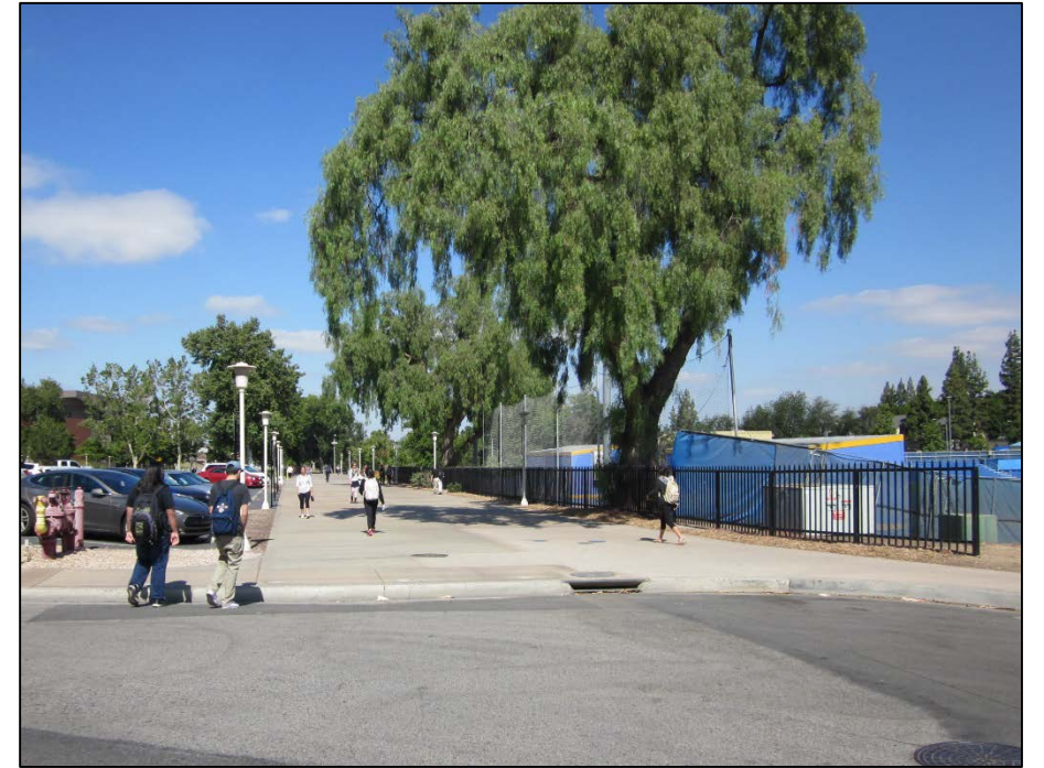
Issue: Disconnected pedestrian path
