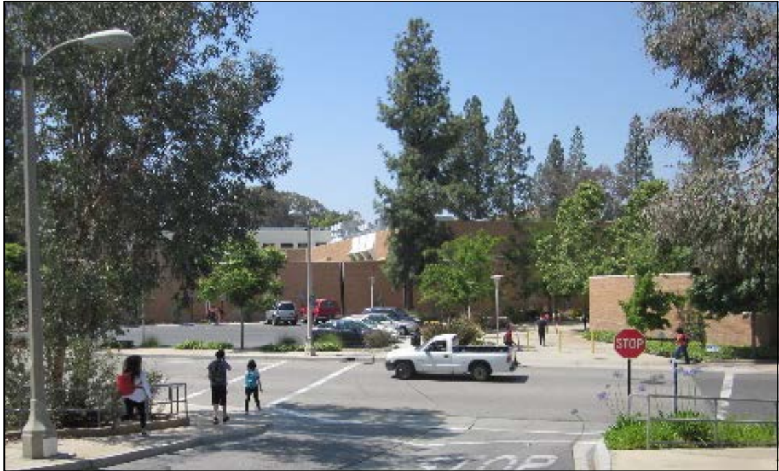
Figure 2.22 – Existing unsafe conditions at intersection with North Campus Drive
