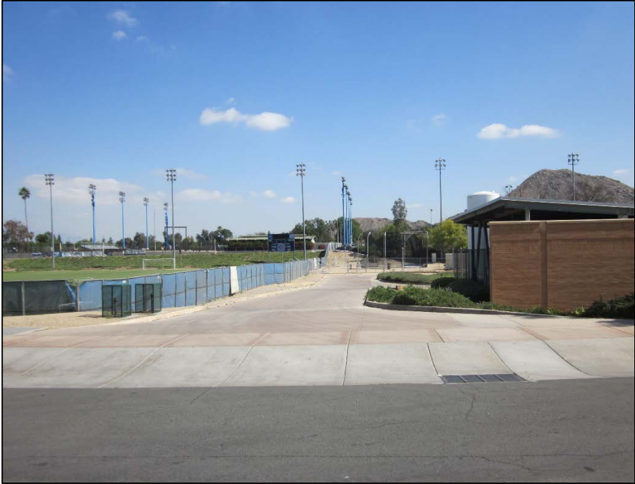
Issue: Disconnected pedestrian path
