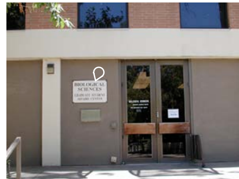
Replace existing sign with W52 Wall Mounted Add W53 Vinyl Letters on Door
