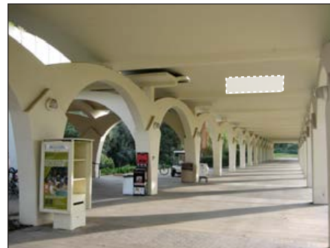
Add W52 Wall Mounted Bldg ID (ceiling hung)
