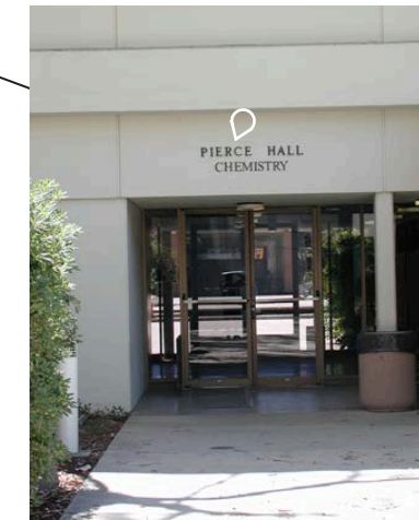
Keep existing sign "Pierce Hall" Remove "Chemistry" Add W53 Vinyl Letters on Door
