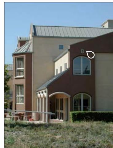
Add W50 Vehicular Bldg ID
