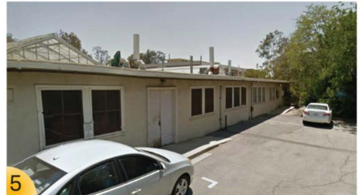
WEST PORTION OF EXISTING HEAD HOUSES AND GREENHOUSES
