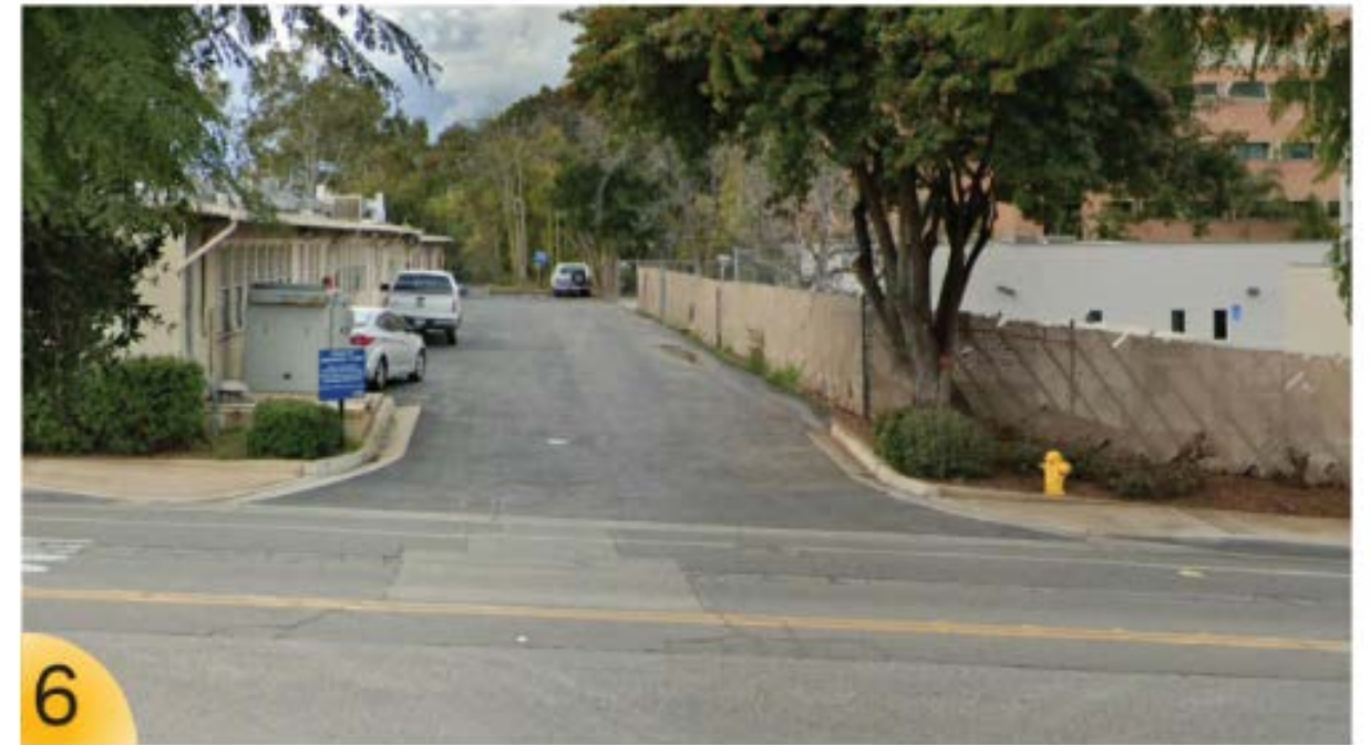
GRADE DIFFERENCE BETWEEN ED2 PROJECT SITE AND HEAD-HOUSE
