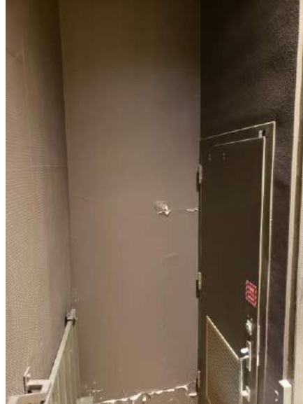
View of Dark Brown Concrete Wall
