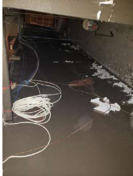
View of Dark Brown Plaster Wall
