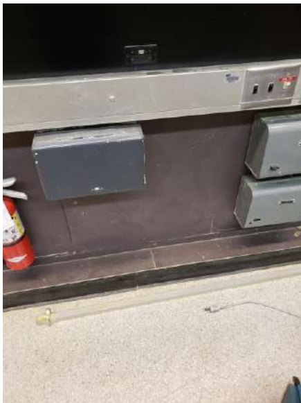
View of Dark Gray Metal Access Panel
