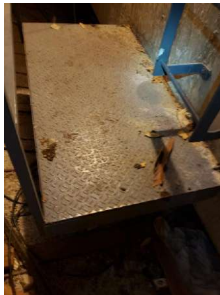
View of Gray Metal Stair Landing
