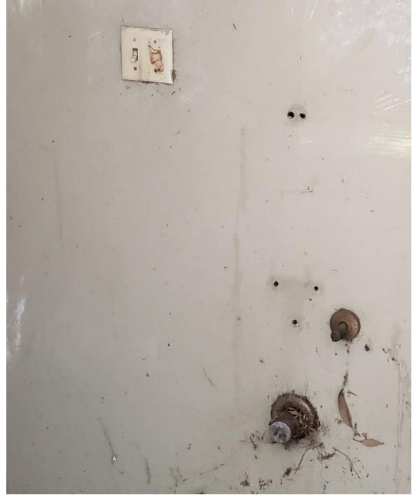
View of Stucco
