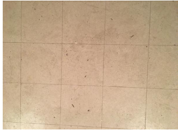
View of 9"x9" Gray Resilient Flooring/Resilient Floor Mastic
