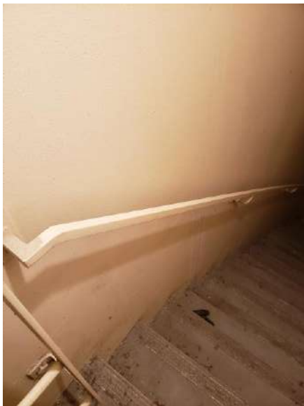
View of Off-White Metal Handrail
