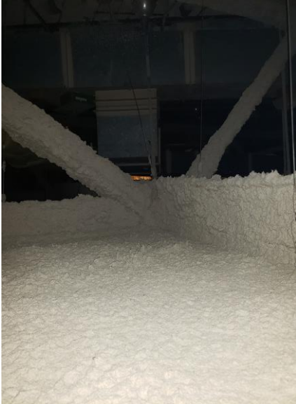
View of Gray Hardpack Fireproofing
