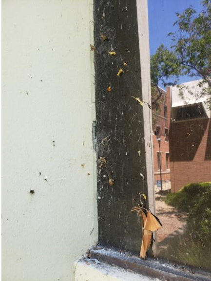
View of Gray Window Putty
