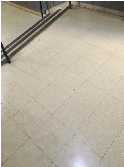
View of 12"x12" Light Tan Resilient Flooring/Resilient Floor Mastic
