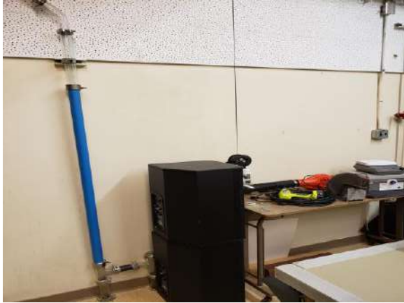
View of Off-White Concrete Wall
