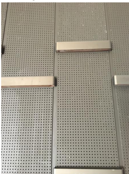
View of 1'x2' Dark Brown Transite Wall Panel
