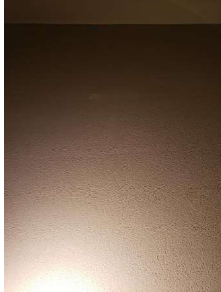
View of Gray Plaster Ceiling
