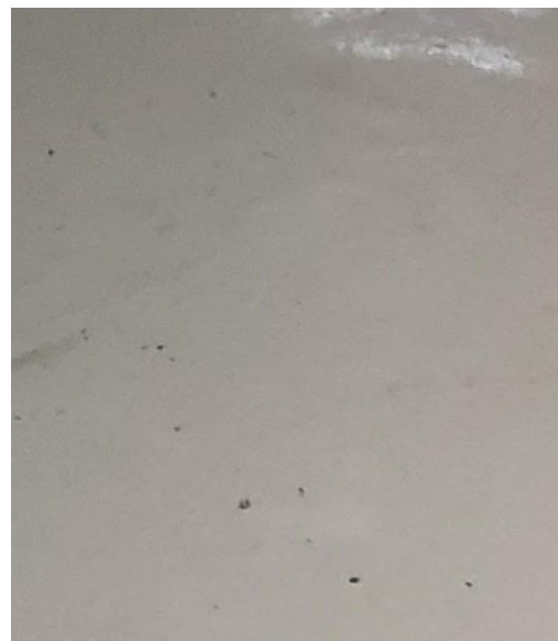
View of Stucco Overhang
