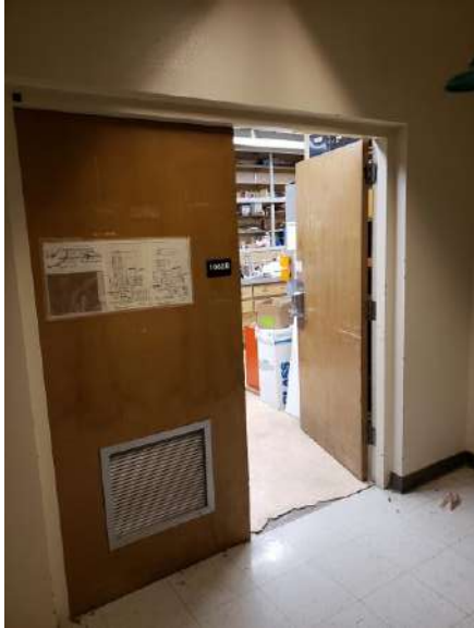
View of Off-White Metal Door Frame
