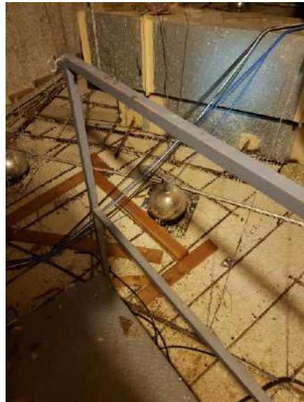
View of Gray Metal Handrail
