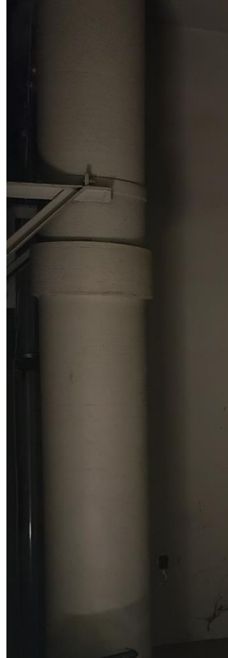
View of 24" Transite Pipe
