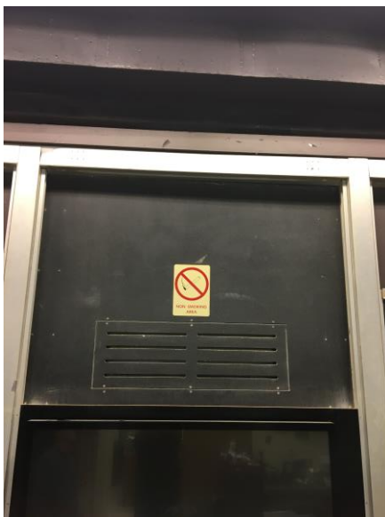
View of Black Transite Wall Panel
