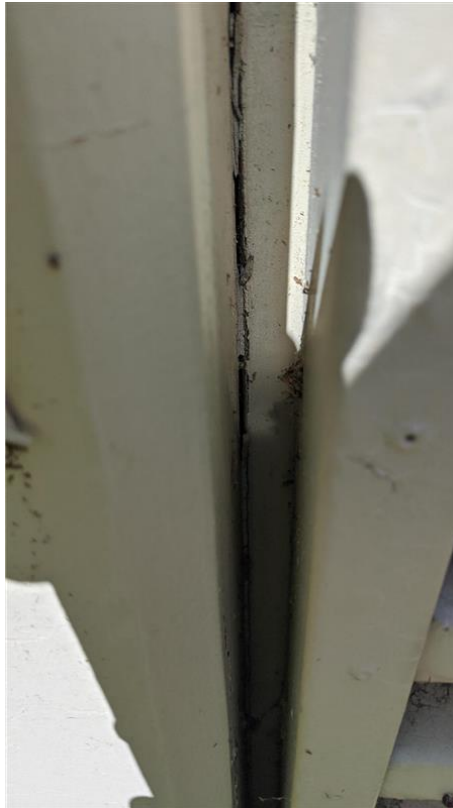
View of Exterior Light Gray Door Frame Caulking
