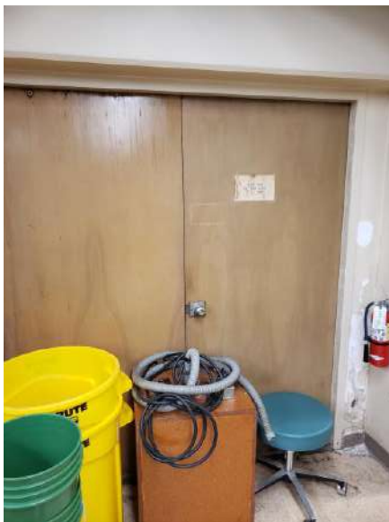
View of Off-White Metal Door Frame
