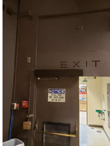
View of Dark Brown Plaster Wall
