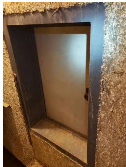
View of Gray Metal Door Frame
