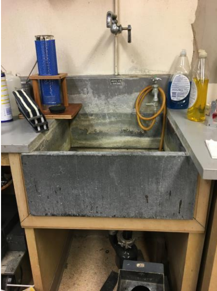
View of Transite Sink
