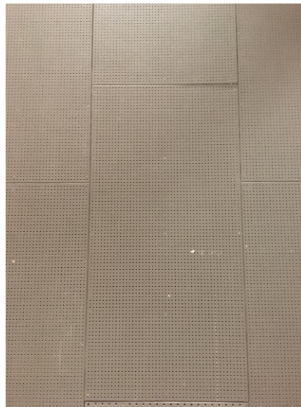
View of 2'x4' Dark Brown Transite Wall Panel
