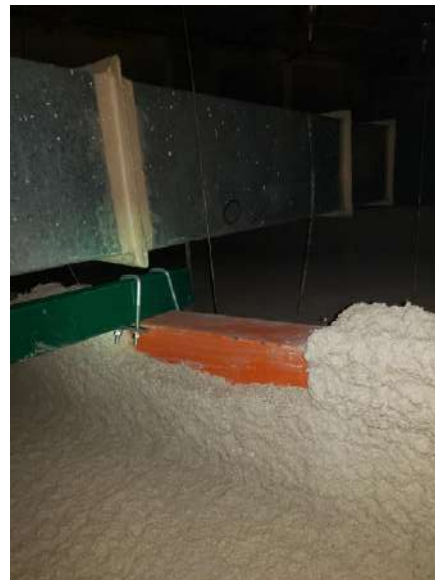
View of Orange Metal Ceiling Beam
