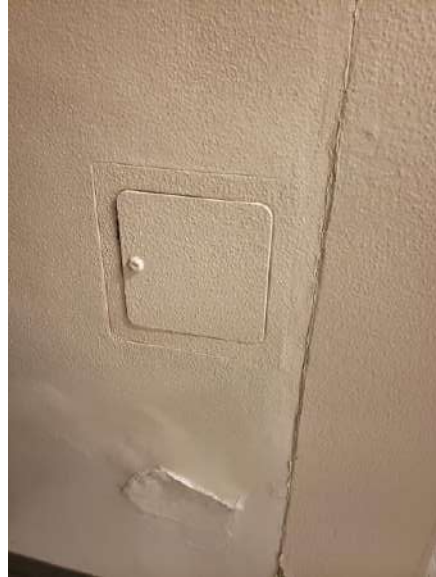
View of Off-White Metal Access Panel
