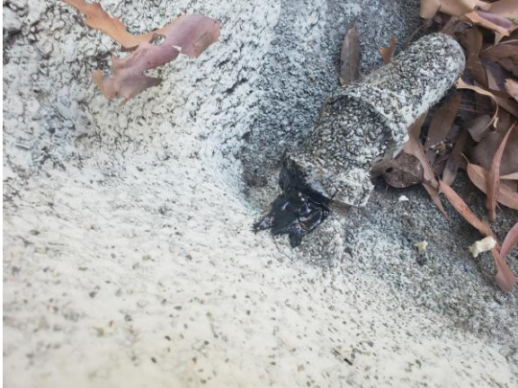
View of Roof Penetration Mastic
