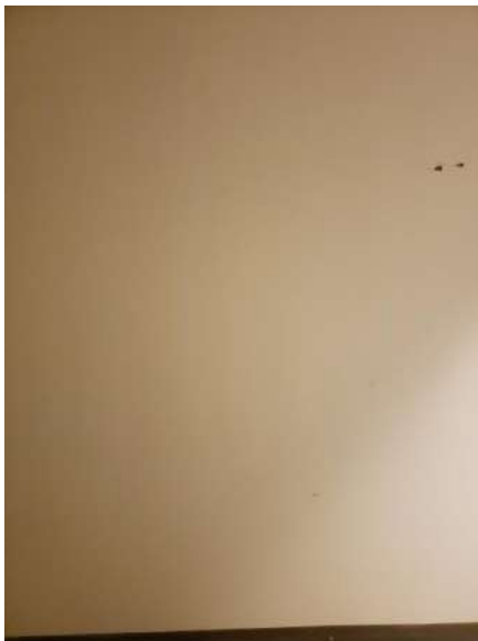
View of Off-White Concrete Wall
