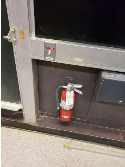
View of Dark Gray Transite Wall
