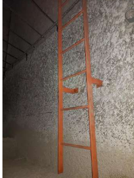
View of Orange Metal Ladder
