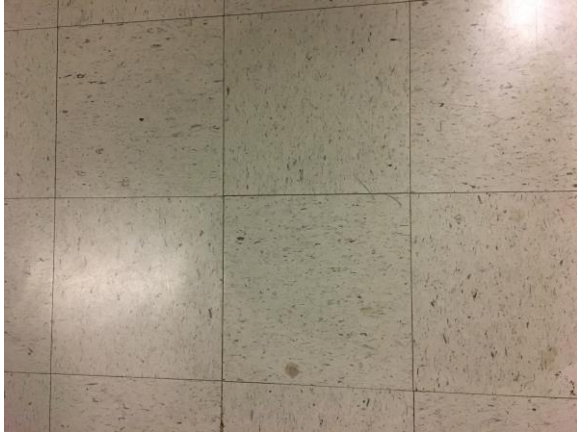
View of 12"x12" Light Gray Speckled Resilient Flooring/Resilient Floor Mastic
