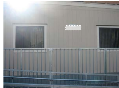
Replace with W52 Wall Mounted Bldg ID
