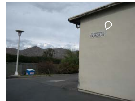
Replace with W52 Wall Mounted Bldg ID
