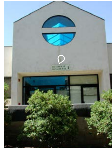
Replace with W52 Wall Mounted Bldg ID
