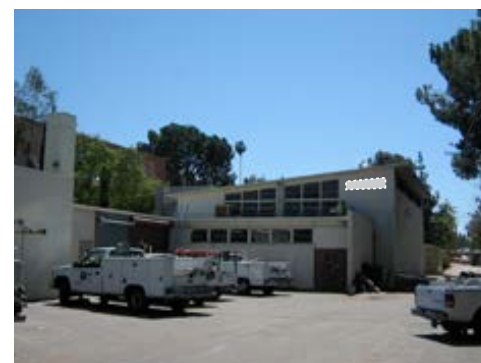
Replace with W54 Parapet Letters
