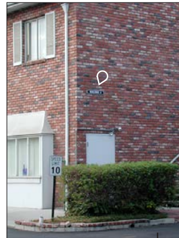
Replace with W52 Wall Mounted Bldg ID
