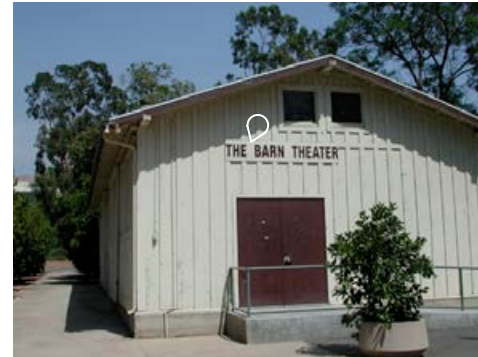
Replace with W52 Wall Mounted Bldg ID
