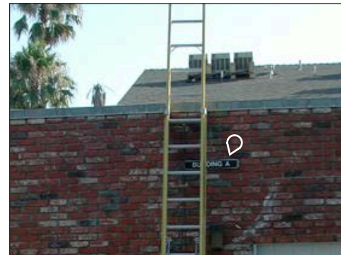
Replace with W52 Wall Mounted Bldg ID
