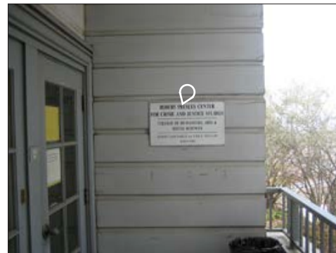
Replace with W52 Wall Mounted Bldg ID
