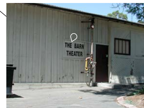
Replace with W52 Wall Mounted Bldg ID
