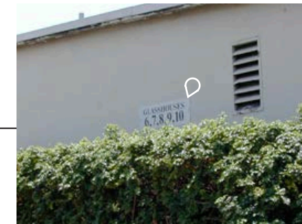
Replace with W52 Wall Mounted Bldg ID
