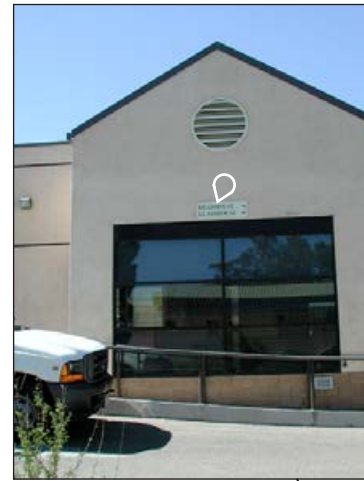
Replace with W52 Wall Mounted Bldg ID
