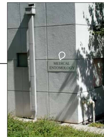
Replace with W52 Wall Mounted Bldg ID
