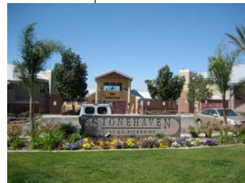
Replace with W50 Vehicular Bldg ID
