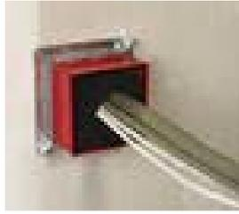
2. Fire Barrier Pass-Through Device 4" Square (UPC # 00051115165979) and Mounting Brackets 4" SQ Single Mounting (Pair) (UPC # 00051115187520)
