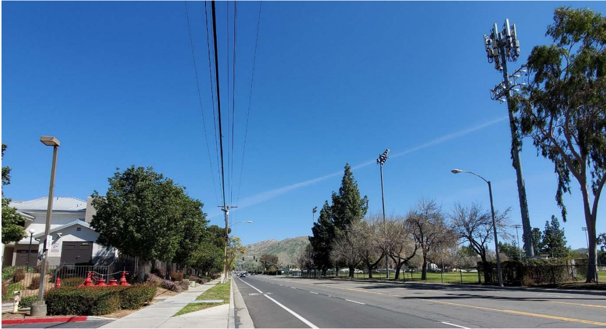
Figure 4.1-36 KVP 3: View East on Blaine Street with Stonehaven Apartments to the Left of Image and the Baseball Field to the Right
