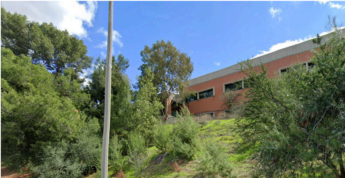
Figure 4.1-29 Salinity Laboratory Viewed from Parking Lot 13 Looking Southeast
