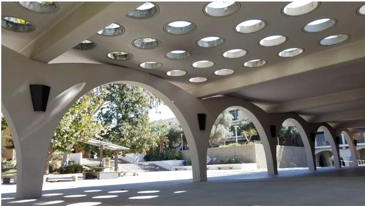
Figure 4.1-21 Arcade Arches to University Theatre Looking Southeast
