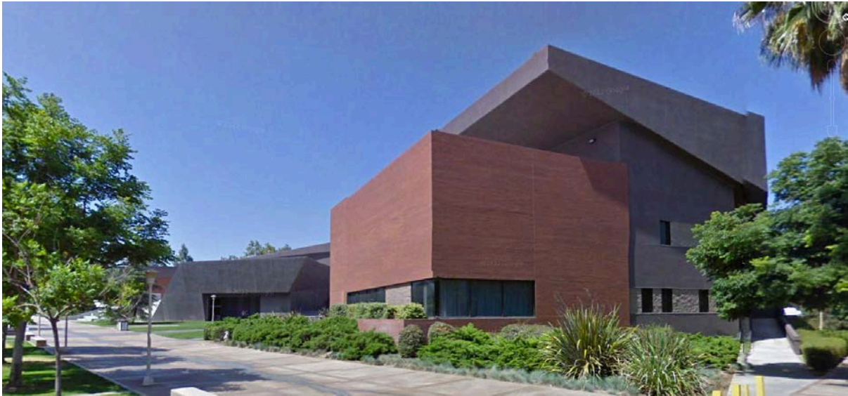
Figure 4.1-14 Arts Building, Looking Southwest
