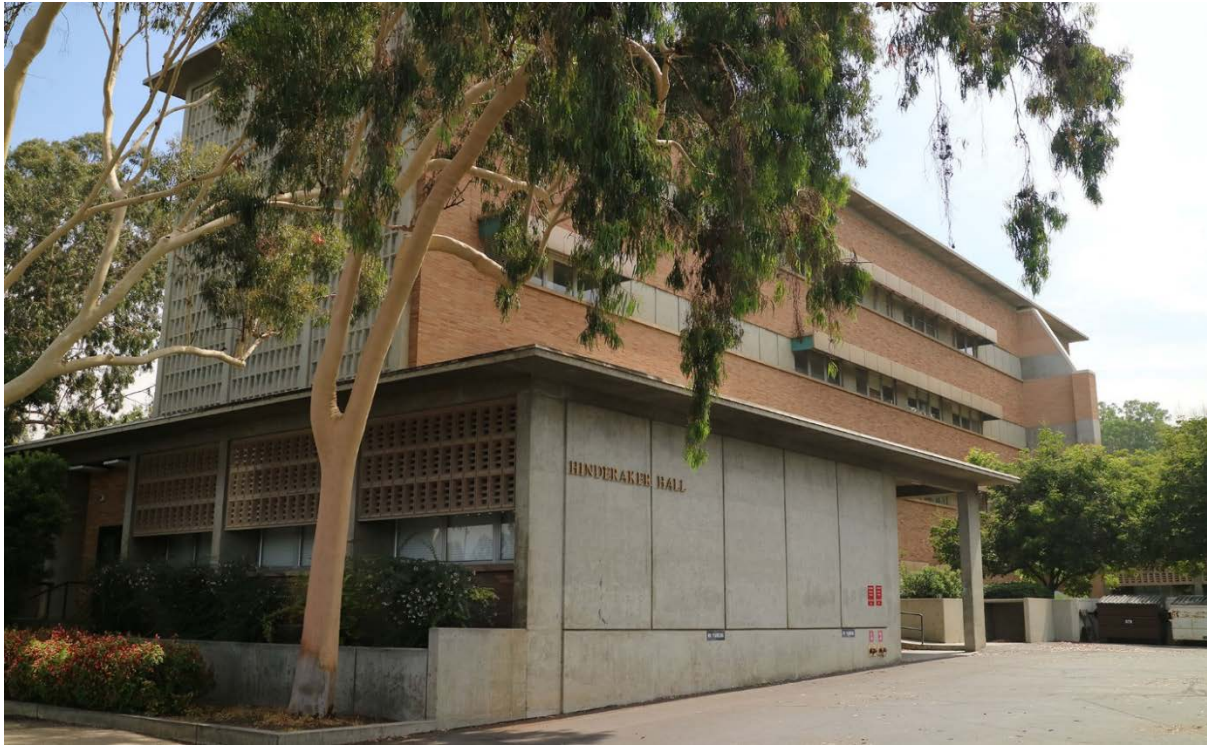
Figure 4.1-12 Hinderaker Hall on the Western Part of East Campus, Looking Northeast
