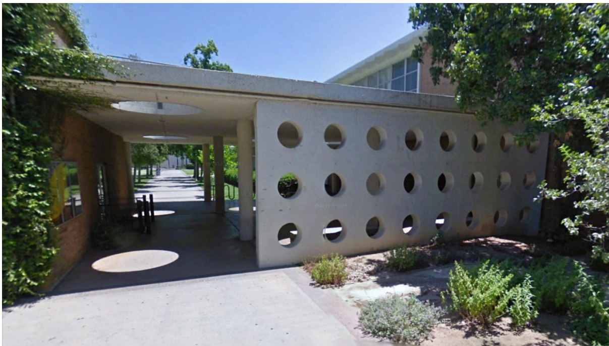
Figure 4.1-22 Watkins Hall Breezeway Looking East
