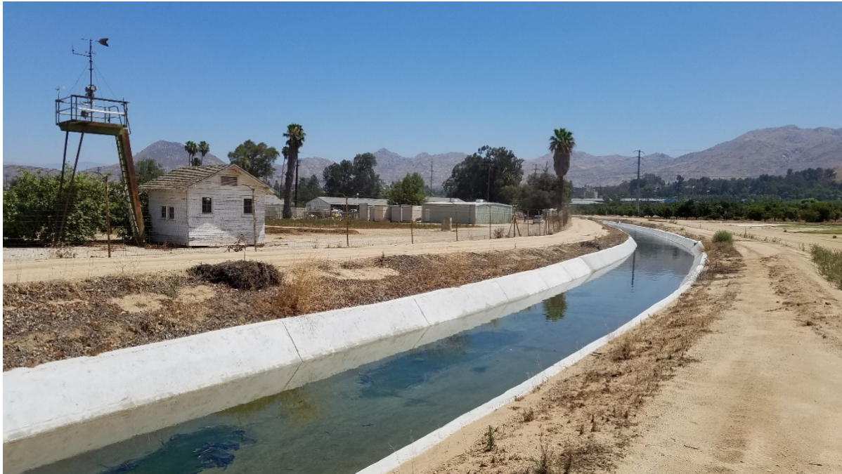
Figure 4.10-5 Gage Canal Looking East in West Campus
