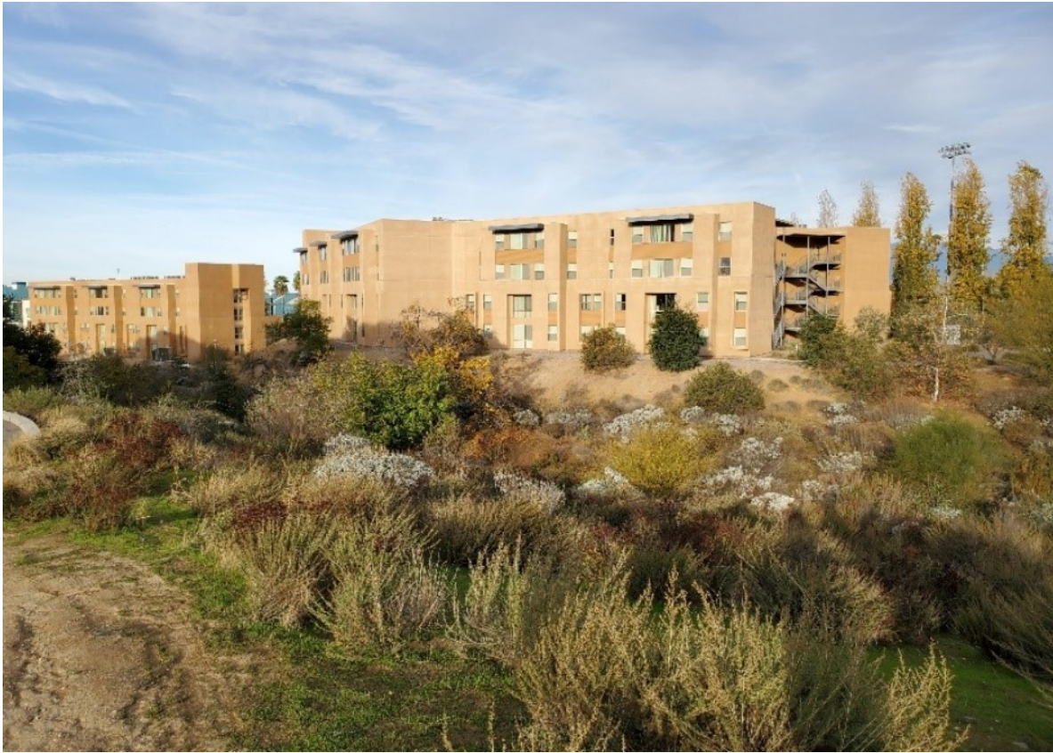
Figure 4.10-3 University Arroyo Tributary Looking Southwest
