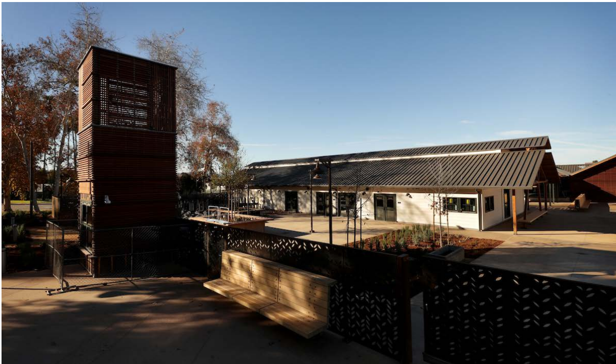
Figure 4.1-15 Renovated Original Structure of The Barn, Looking Southwest
