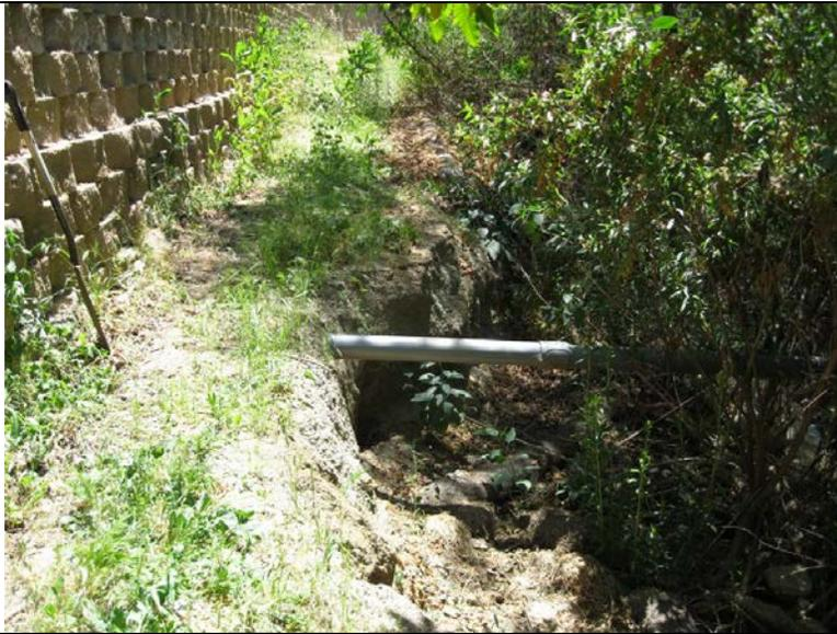
Photograph 4 Undercutting of slope by stream flows along eastern bank, immediately adjacent to retaining wall.
