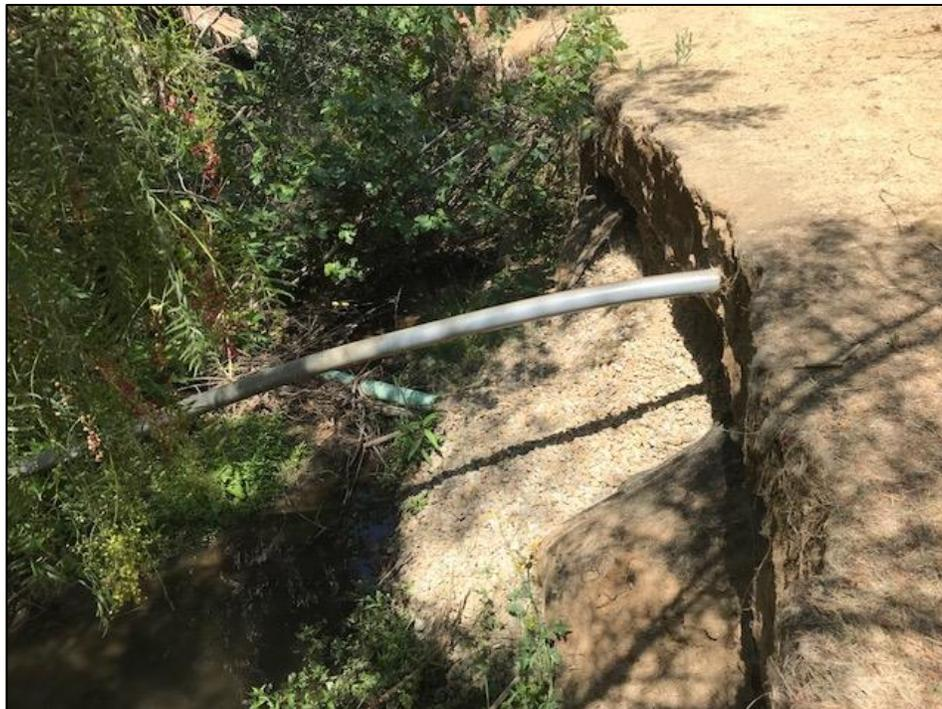
**Photo 3.** View of the banks of the streambed with severe erosion adjacent to the upper terrace. The image depicts a drainage pipe and crushed rock fill where the bank has eroded.
