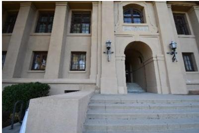
Rectangular wood casement windows with larger windows with transoms at second floor at primary elevation
