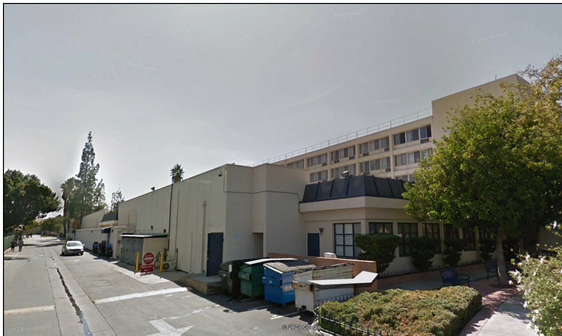
Figure 6. North end of east elevation, view southeast (Google Earth)
