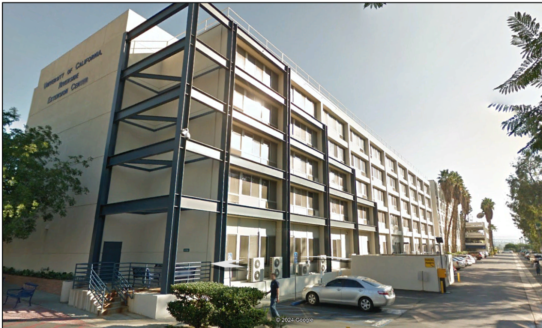
Figure 2. West elevation, view southeast (Google Earth)
