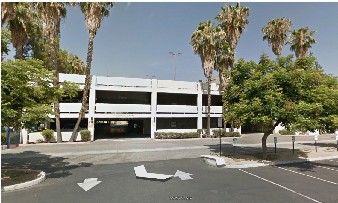
Figure 4. South end of east elevation, view west (Google Earth)
