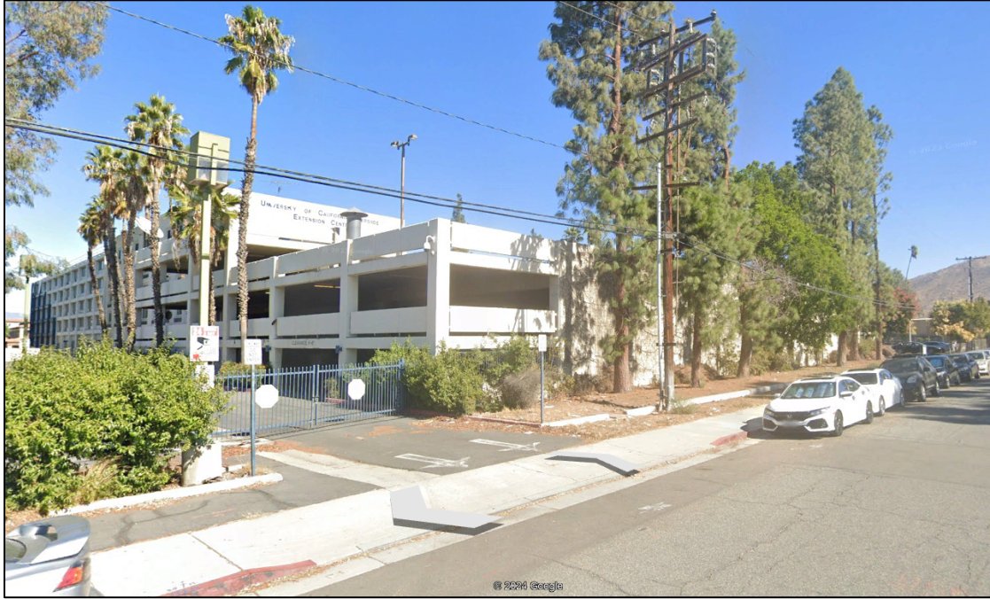
Figure 3. West and south elevations, view northeast (Google Earth)
