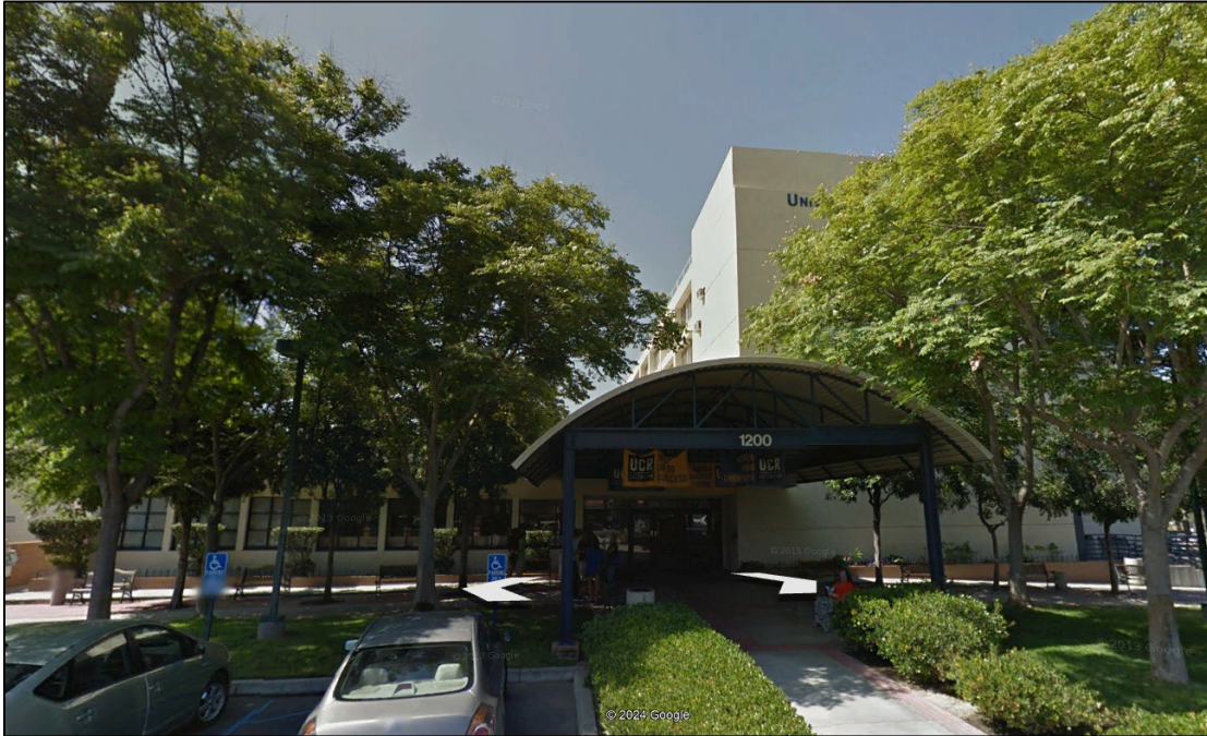
Figure 1. Overview of north (primary) façade, view south (Google Earth)
