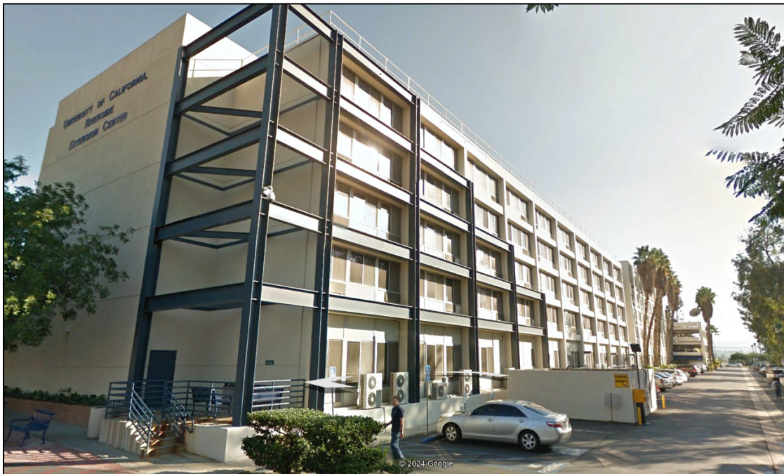
Figure 2. West elevation, view southeast (Google Earth)
