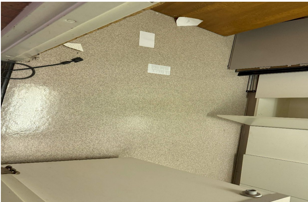
Photograph 12: Beige pebble pattern sheet flooring on concrete, room 383-non-asbestos.
