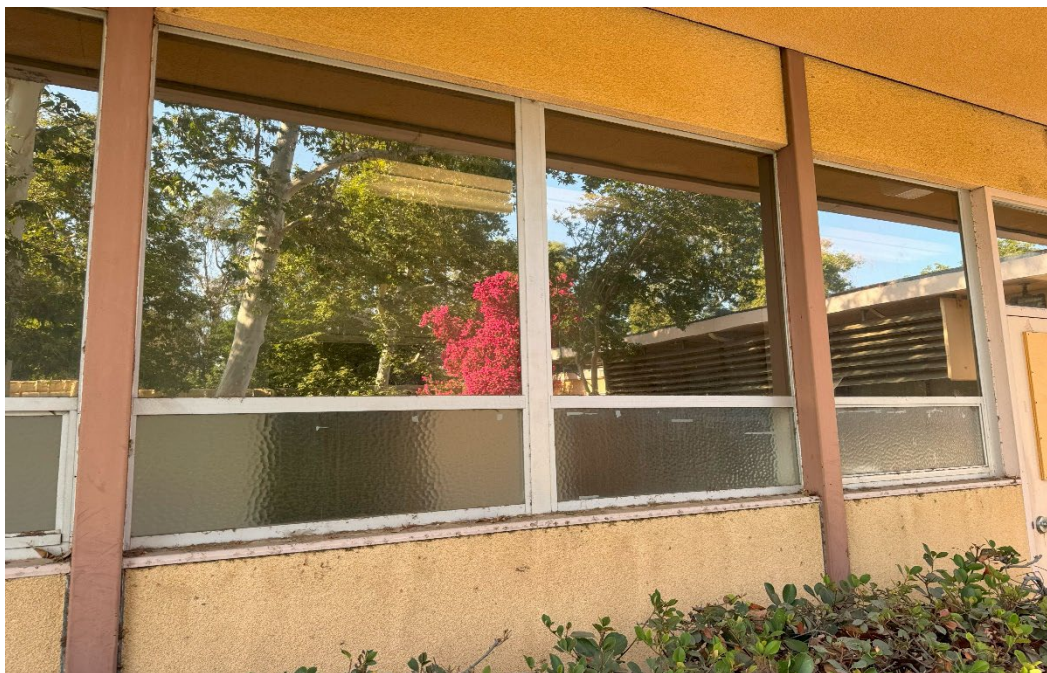
Photograph 1: Metal wall posts-paint negative for lead, stucco ACCM by Point Count.
