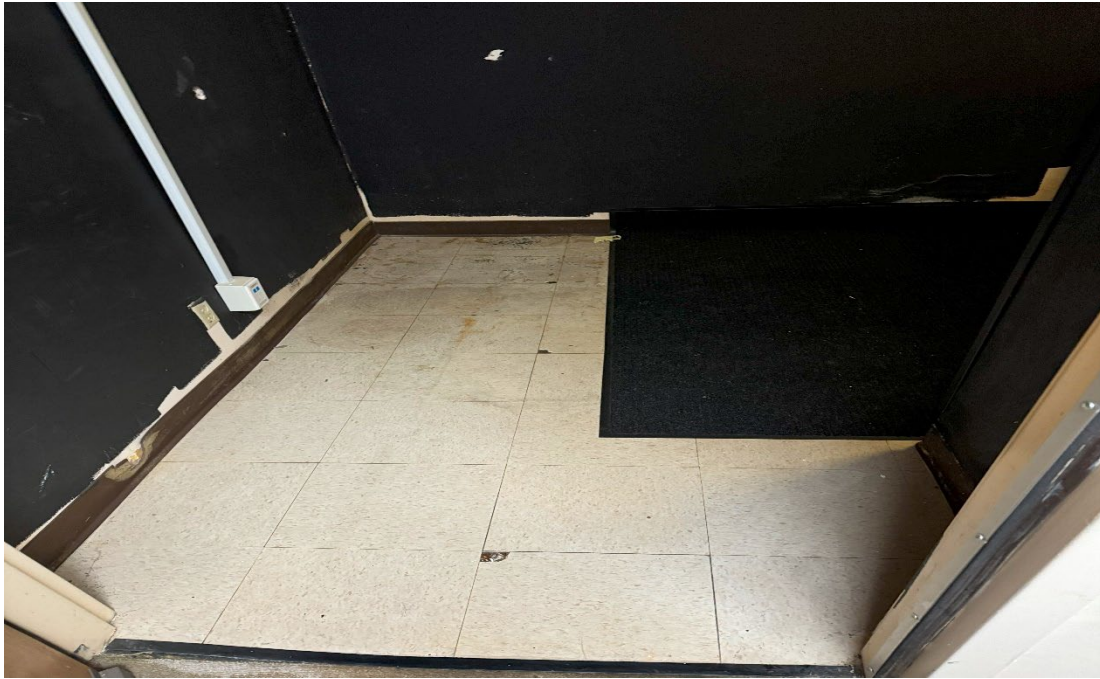
Photograph 9: Room 128 B, asbestos containing 12"x12" Off White VFT with mastic on concrete.
