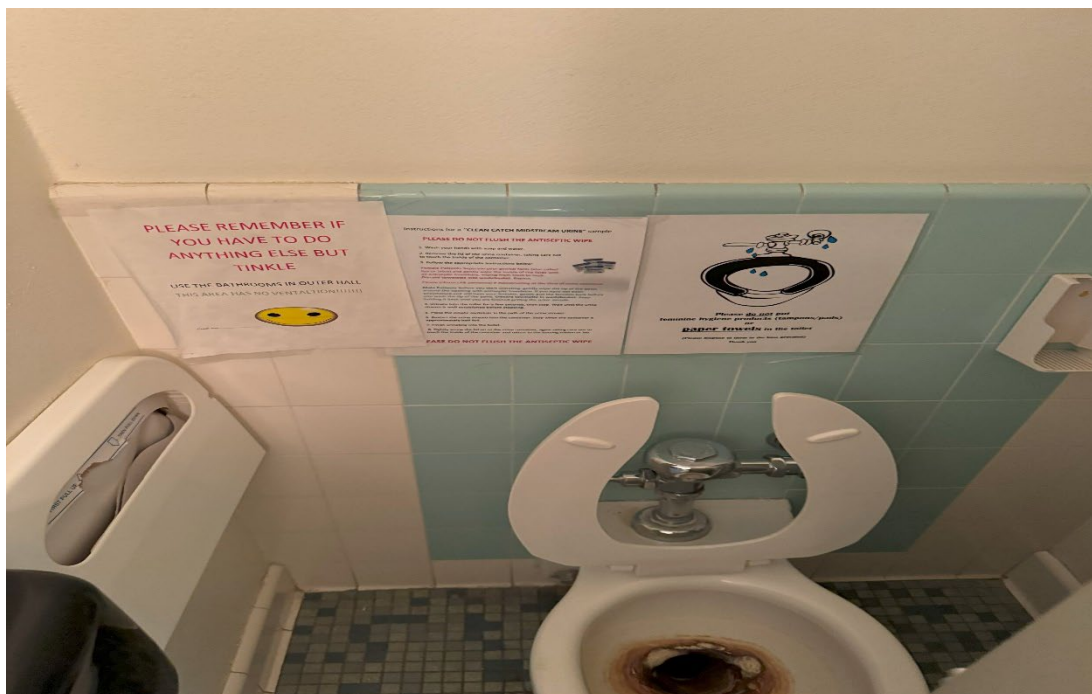
Photograph 23: Lead containing wall and cove base ceramic tiles at restrooms.
