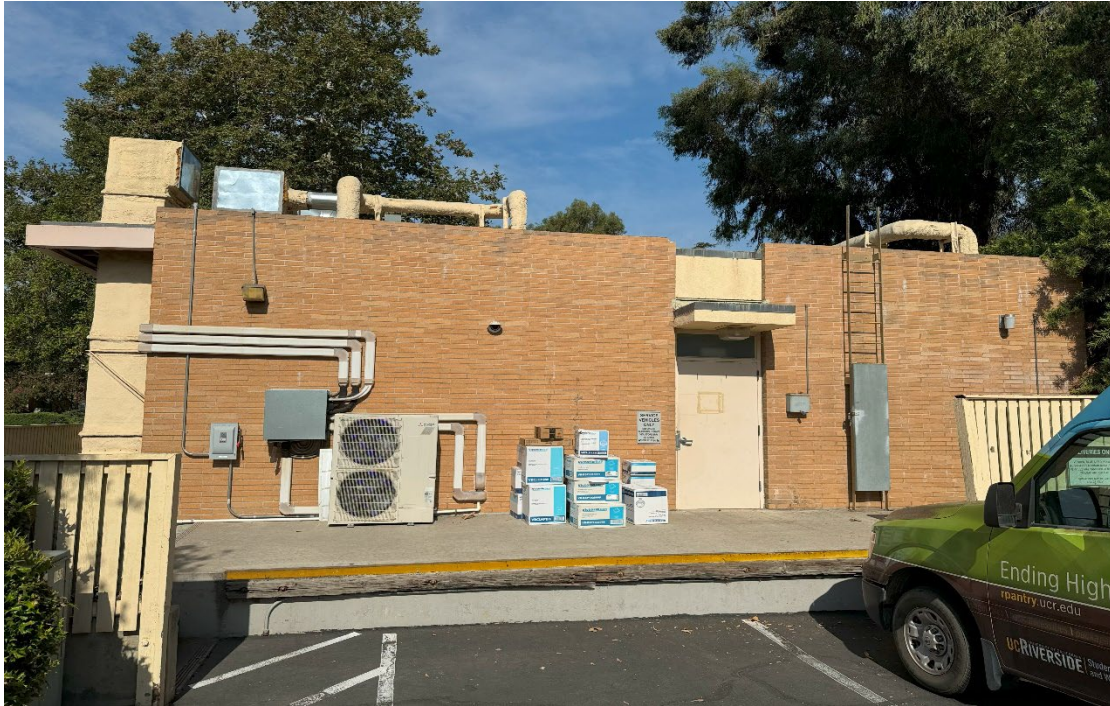
Photograph 21: Yellow Lead base paint on loading dock edge bumper/Intact.
