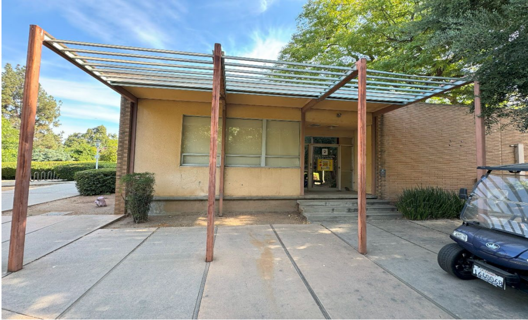
Photograph 19: Brown sunshade support posts with lead base paint-exterior southwest-SW entry.
