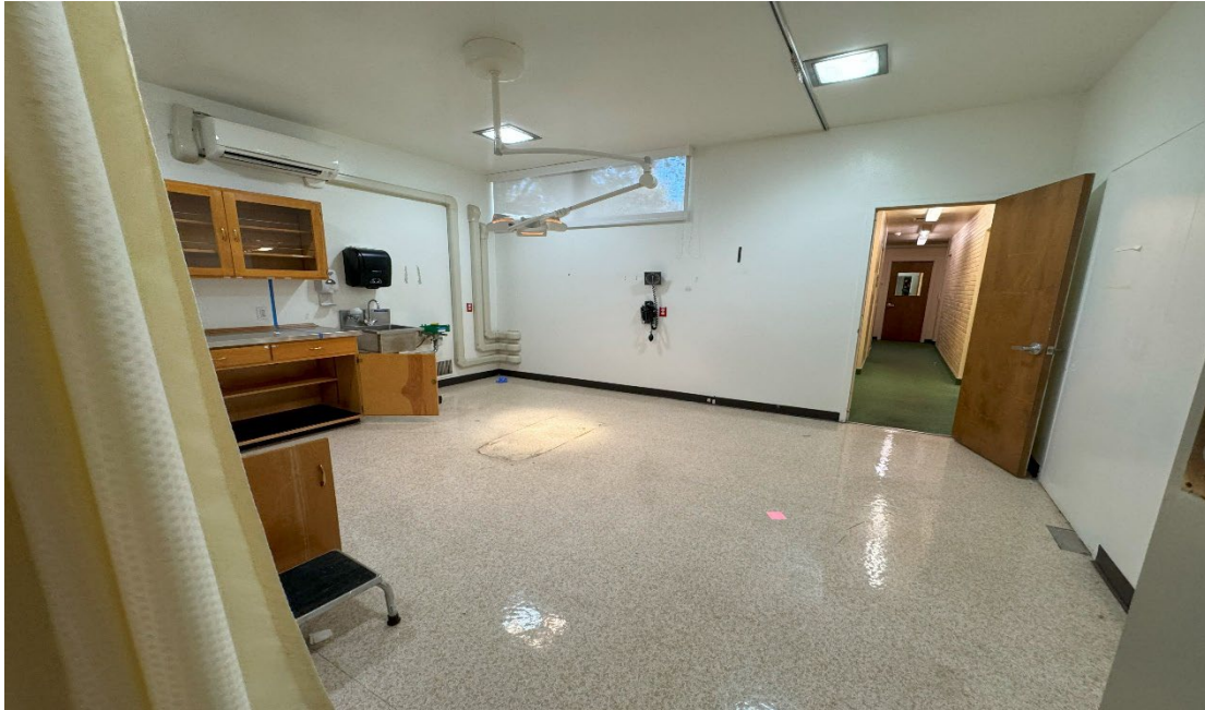
Photograph 5: Rm 207, Asbestos containing sheet flooring, cove base is ACCM.
