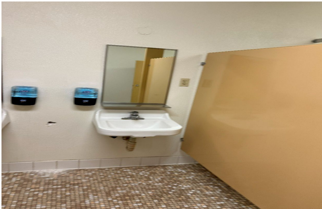
Photograph 10: Northeast restrooms-ceramic cove base and flooring-non lead containing. walls/ceilings are accm.
