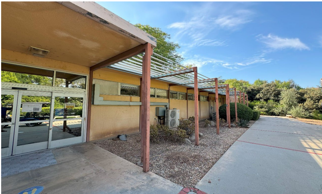
Photograph 20: Brown sunshade support posts with lead base paint-west entry.
