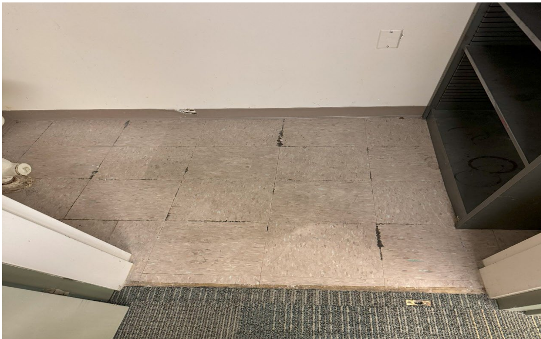
Photograph 5: Rm 207, Asbestos containing sheet flooring, cove base is ACCM.
