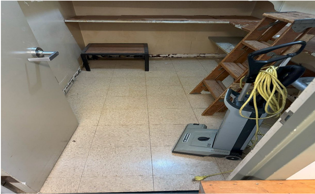
Photograph 7: Room 305, asbestos 12"x12" beige VFT with mastic on concrete.
