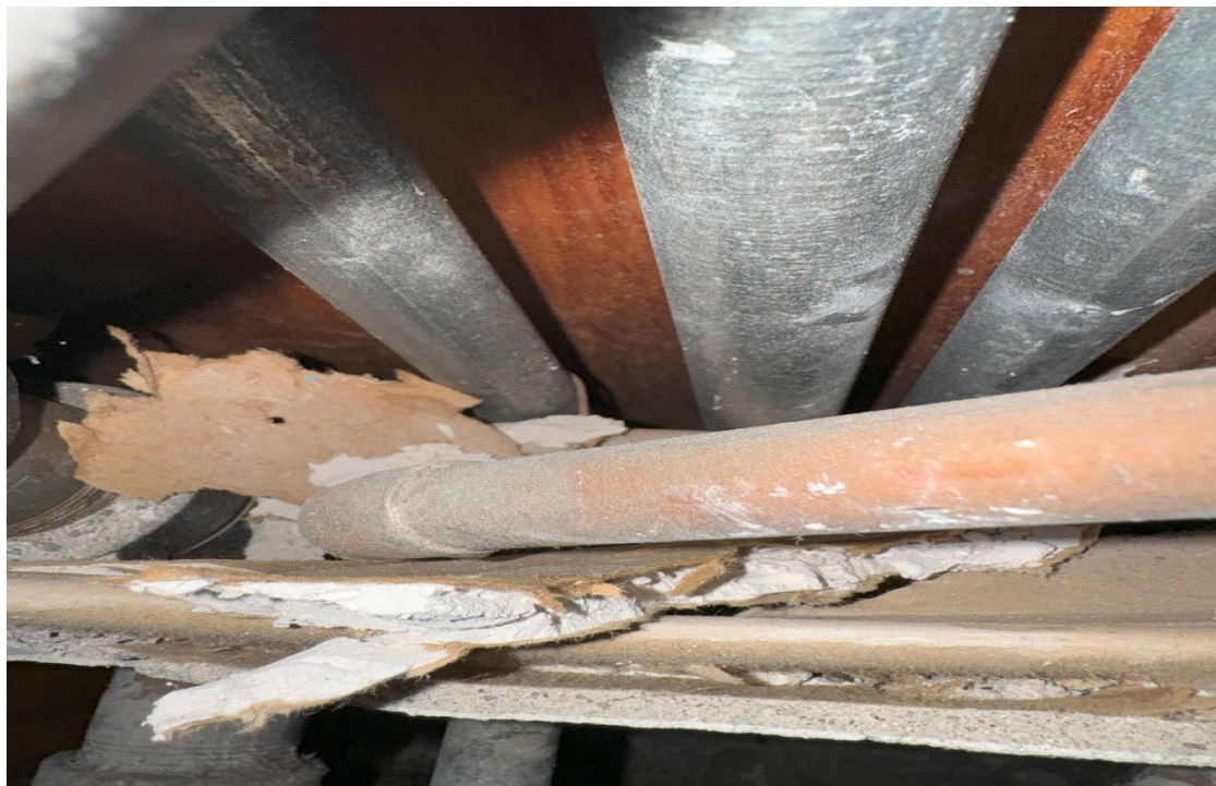
Photograph 15: Fiberglass pipe insulation in wall cavity, restroom 397
