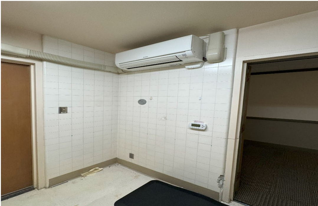
Photograph 7: Room 305, asbestos 12"x12" beige VFT with mastic on concrete.
