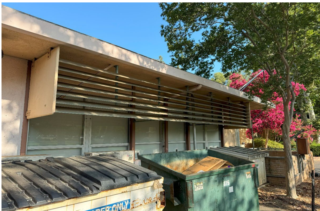
Photograph 2: Concrete louver side supports, non-acm, no LBP
