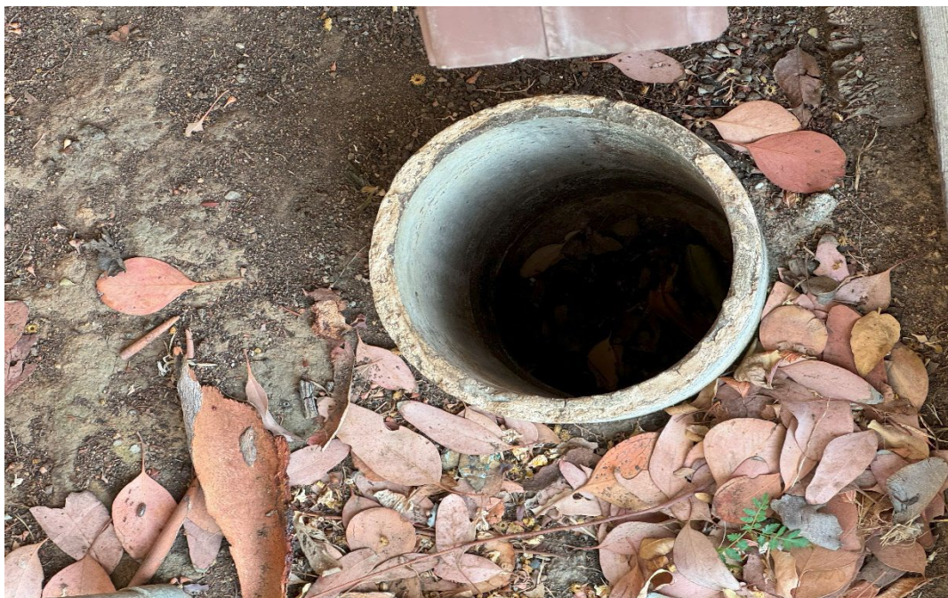
Photograph 3: 8" Asbestos transite pipe-southeast of south wing and northwest of building.
