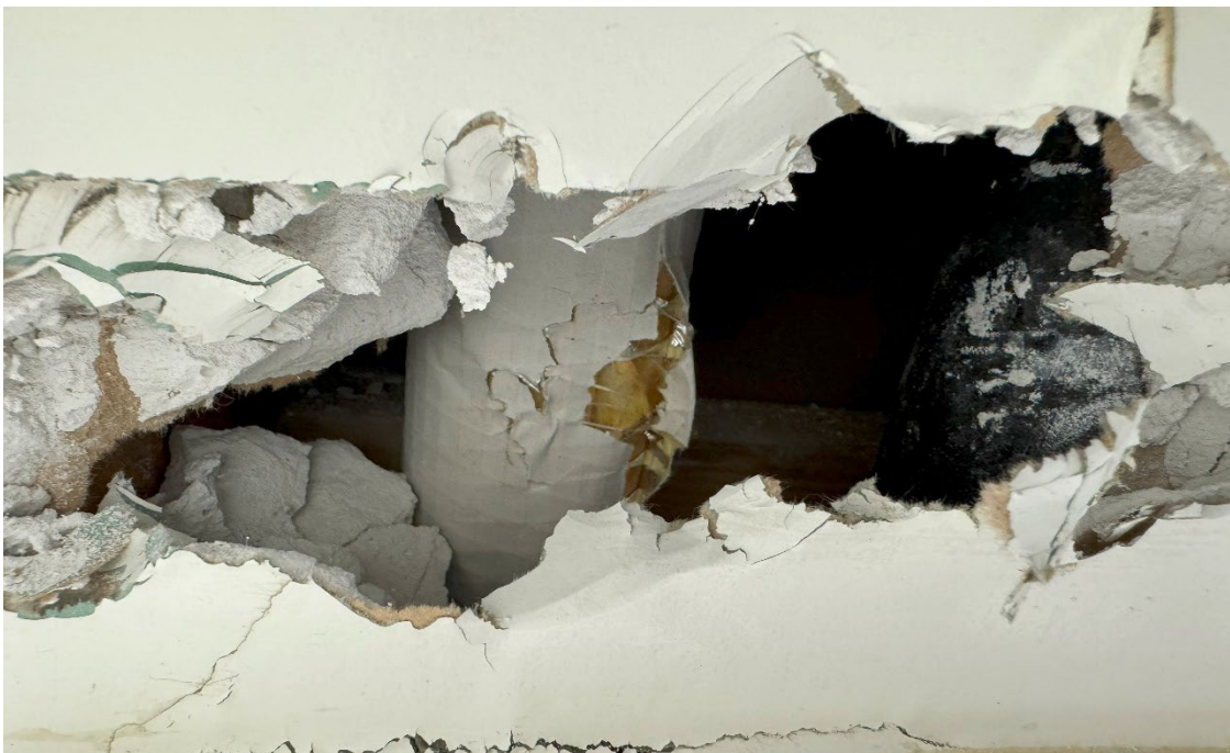
Photograph 15: Fiberglass pipe insulation in wall cavity, restroom 397
