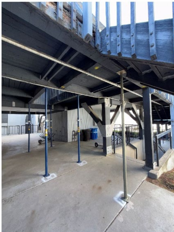
Photograph 5: Bannockburn Village, metal support poles located beneath walkways
