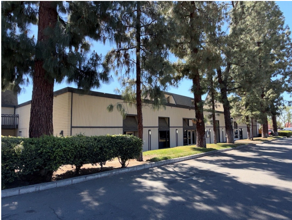
Exhibit 3. Bannockburn Village support building, view southwest
