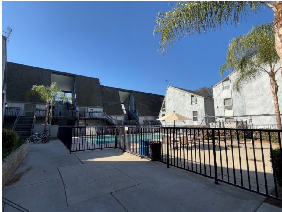
Photograph 2: Bannockburn Village, view southwest
