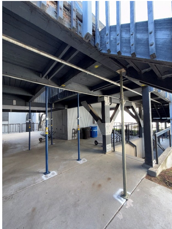
Exhibit 5. Bannockburn Village, metal support poles located beneath walkways.
