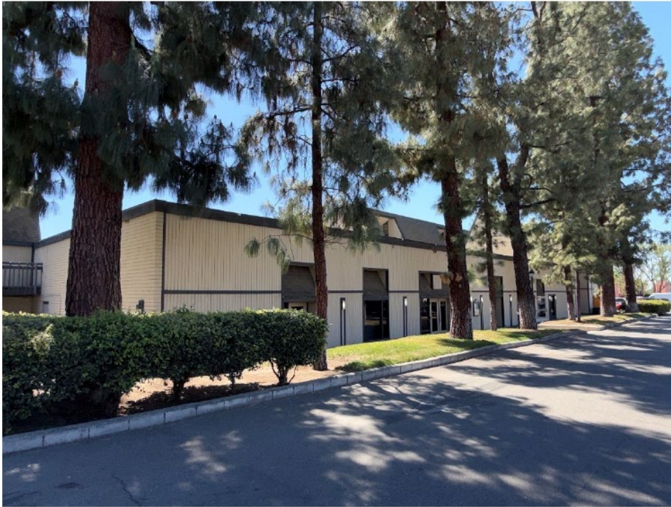
Photograph 3: Bannockburn Village Support Building, view southwest
