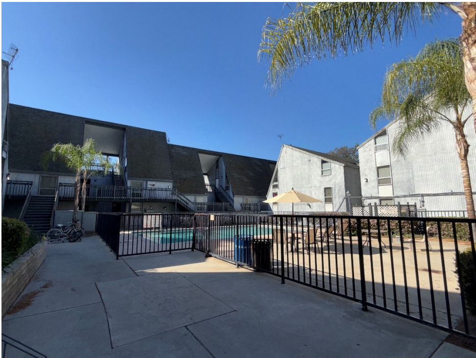
Photograph 3. Bannockburn Village, view southwest
