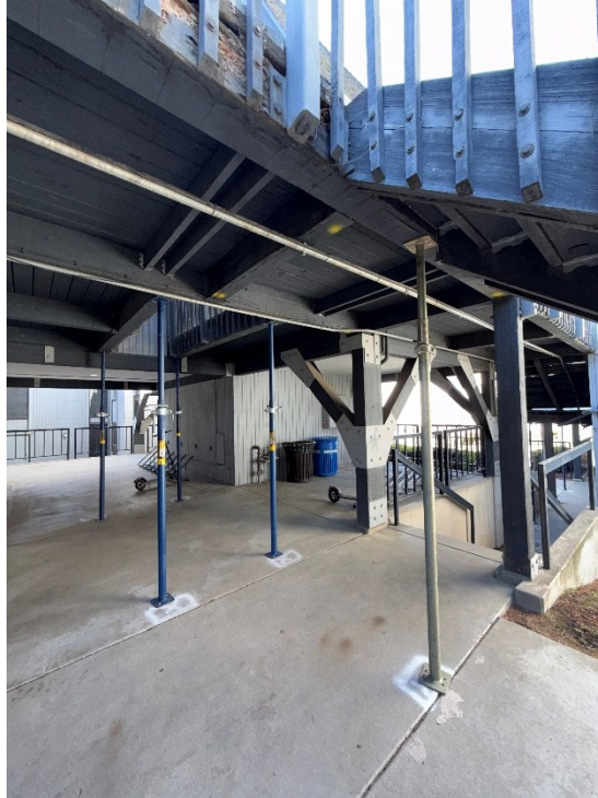
Photograph 6. Bannockburn Village, metal support poles located beneath walkways.
