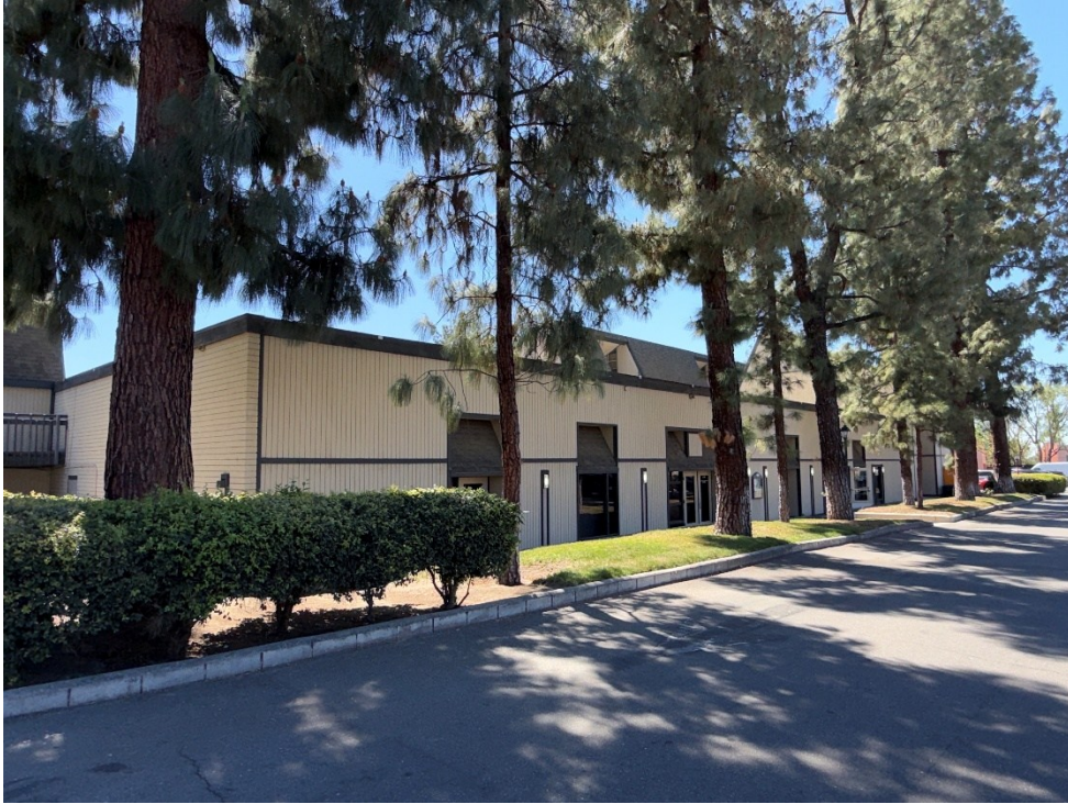
Photograph 4. Bannockburn Village support building, view southwest
