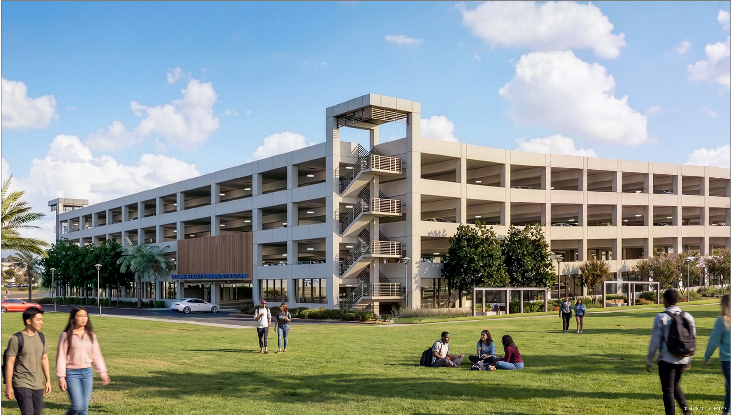
Figure 2-12 Blaine Street Parking Structure Conceptual Rendering Looking North Towards Parking Structure
