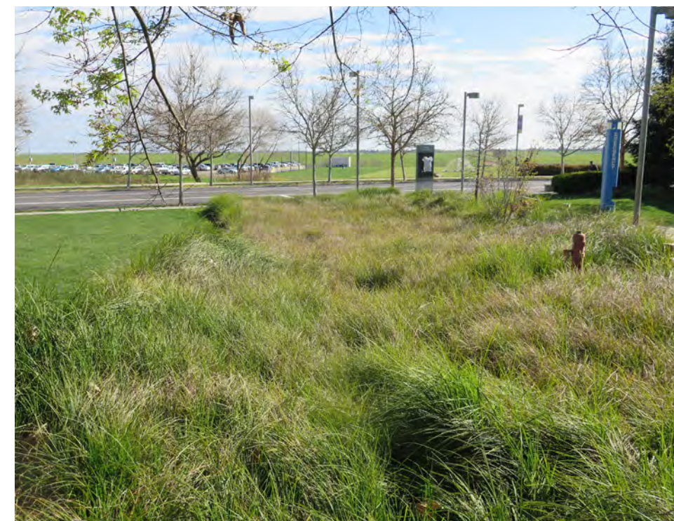
Stormwater swale, UC Merced
