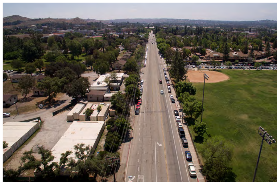
Canyon Crest Drive north of Linden, today
