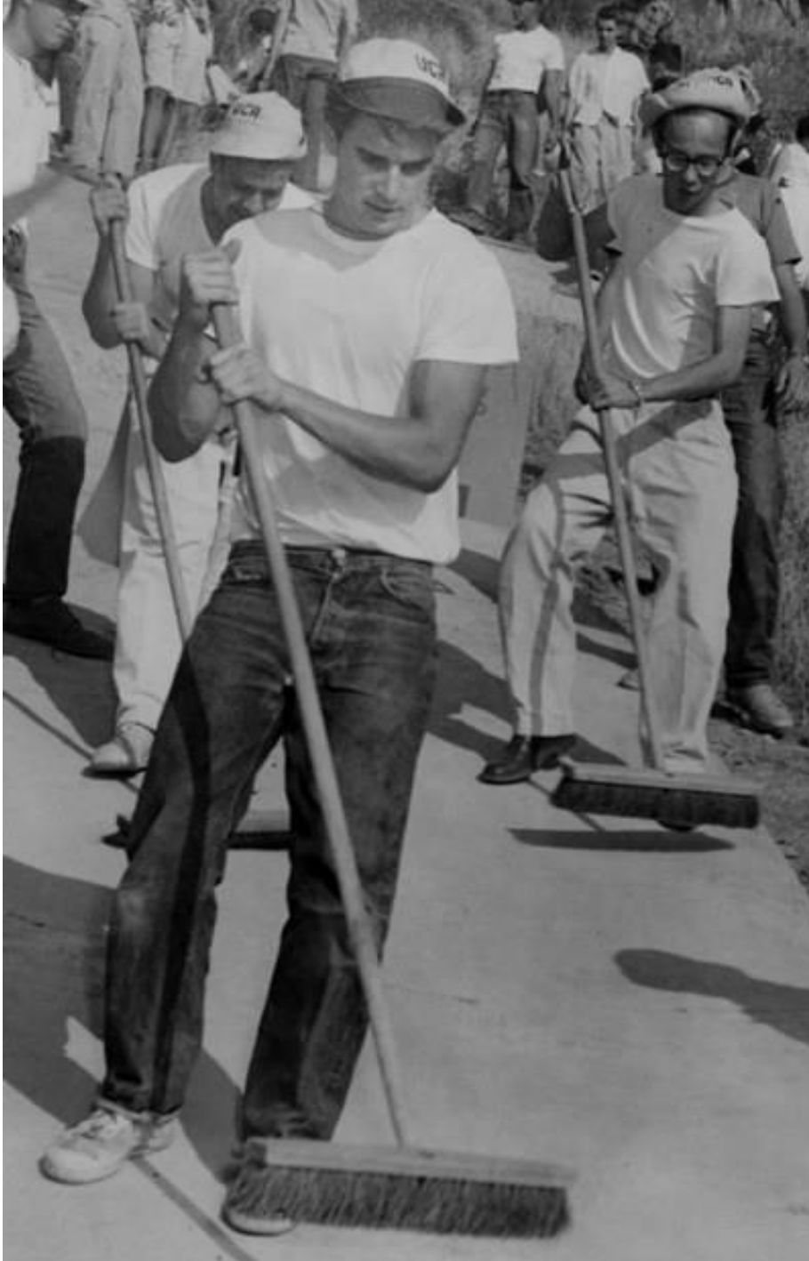
Figure 26 Construction of UC "C", c. 1955
