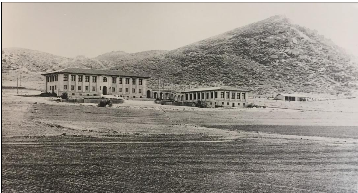
Figure 9 Horticulture Building (Anderson Hall 1), 1916 (left) and Irrigation Building (Anderson Hall 2), 1916 (right), prior to 1931 addition of Soils/Plant Nutrition Wing (Chapman Hall)
