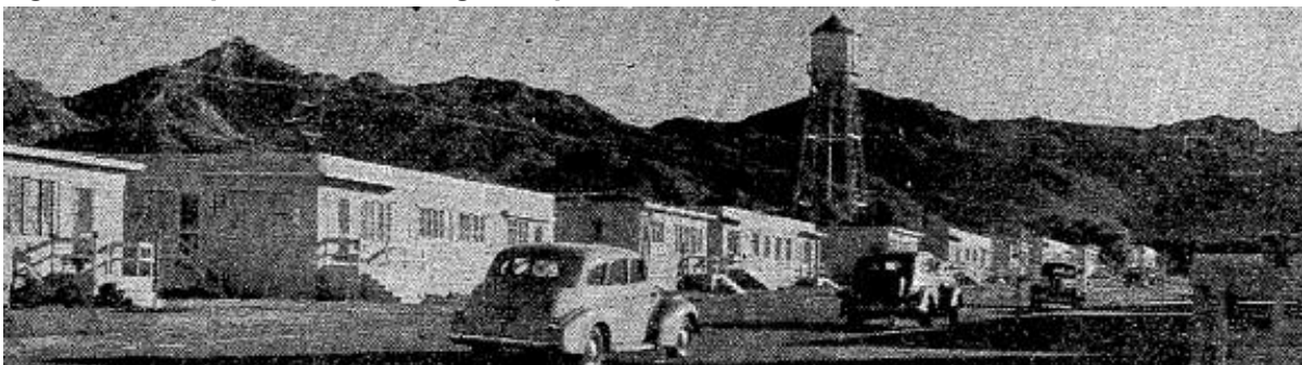
Figure 32 Canyon Crest Housing Complex, 1943
