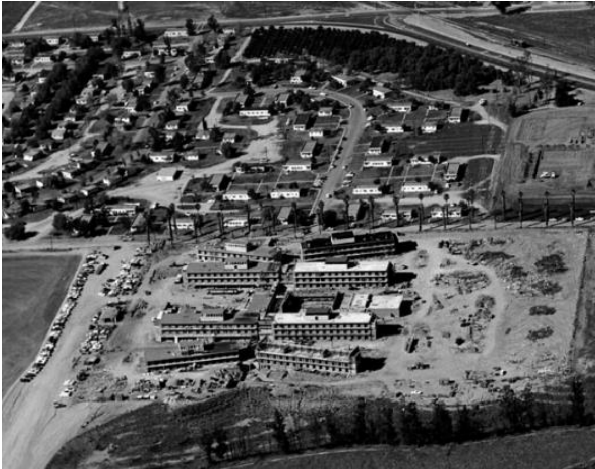
Figure 34 Aerial View of Aberdeen-Inverness Residence Hall Under Construction, c. 1959
