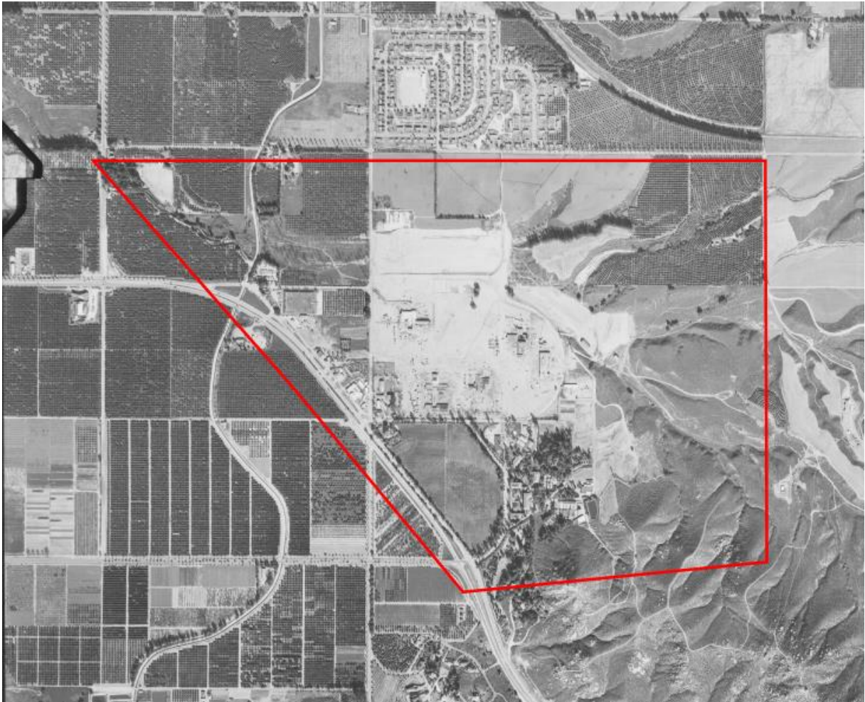
Figure 17 Aerial Photograph of UCR and Surrounding Vicinity, 1953
