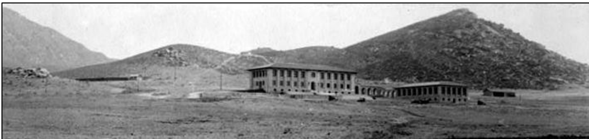
Figure 51 Overview of the Citrus Experiment Station; a third addition (Soils/Plant Nutrition Wing [now Chapman Hall]) was constructed in 1931 to form the current U-shaped complex
