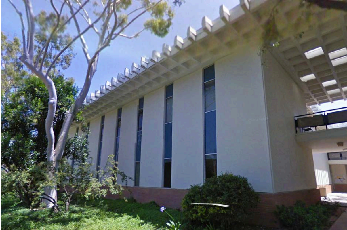
Figure 4.1-19 West Side of Sproul Hall Looking Northeast
