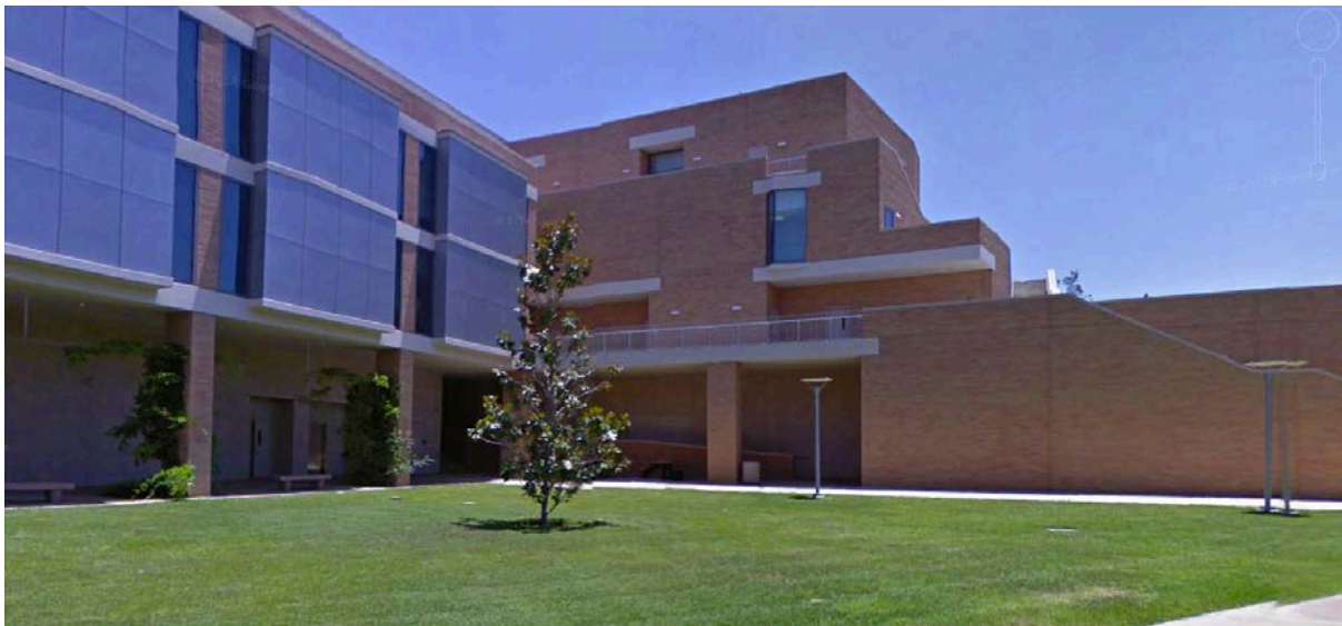
Figure 4.1-13 CHASS Interdisciplinary Building, Looking Northeast
